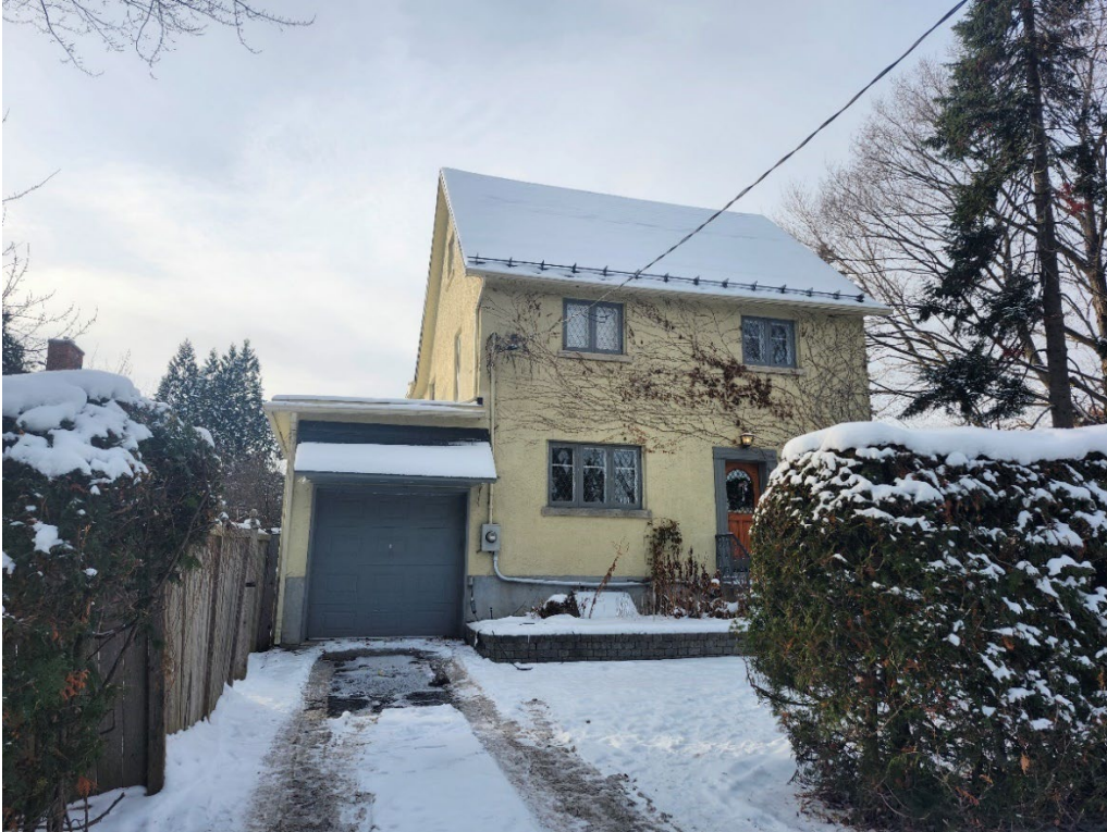
East elevation of building as seen from Springfield Road.
