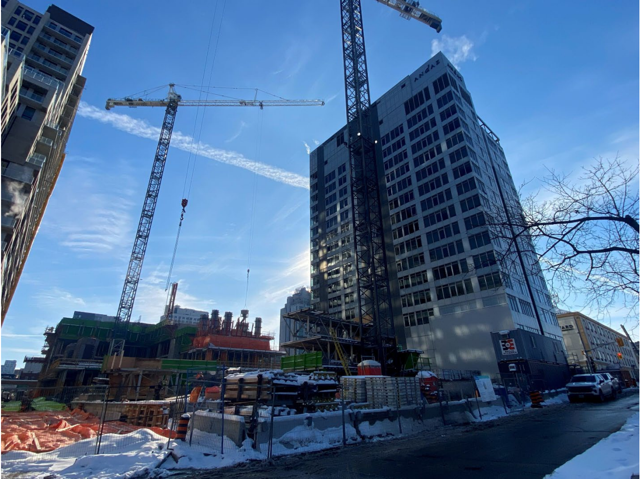
Image showing the subject site at 110-116 York Street, looking south west.
