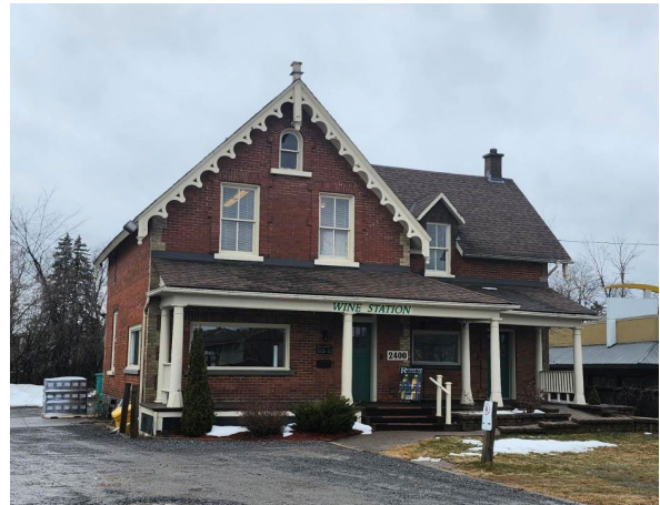
Front street facing/east façade, Source: City of Ottawa, 2025
