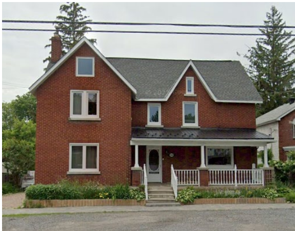
3560 Albion Road, built circa 1860, Ward 10, Source: Google Streetview, 2021
