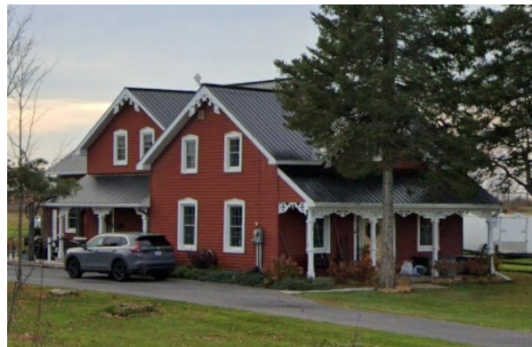
4538 High Road, built circa 1855, Ward 22, Source: Google Streetview, 2024
