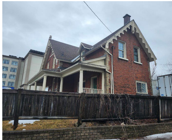
North façade, Source: City of Ottawa, 2025
