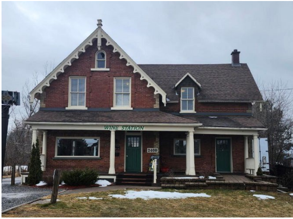
Front street facing/east façade, Source: City of Ottawa, 2025
