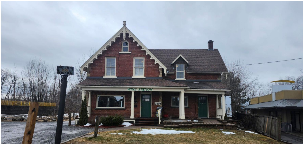
2400 Bank Street, front façade, Source: City of Ottawa Staff, 2025
