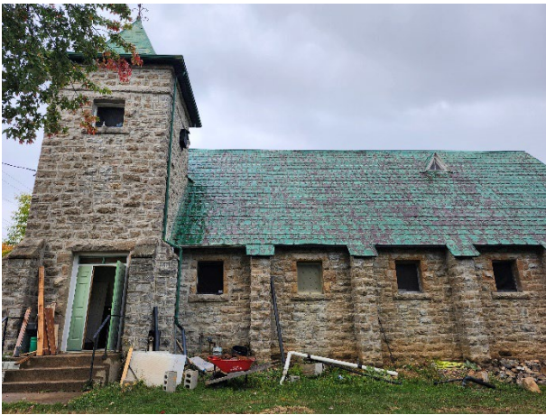
South elevation with main entrance through tower. Source: City of Ottawa, 2025.
