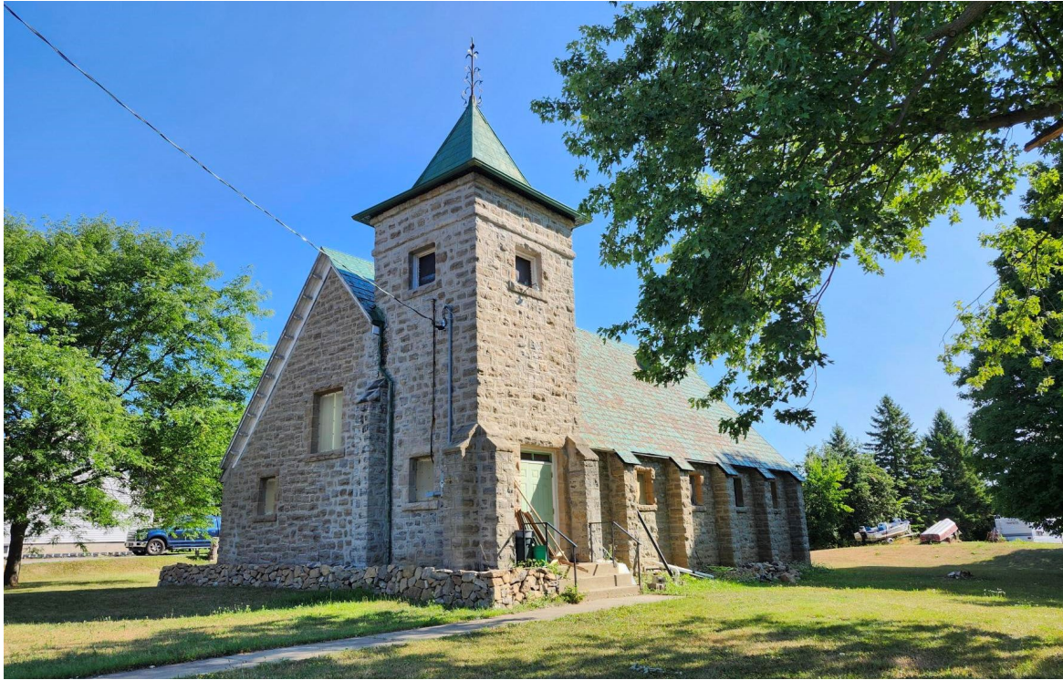
Front (west) façade facing Bank Street. (Source: City of Ottawa, 2025)
