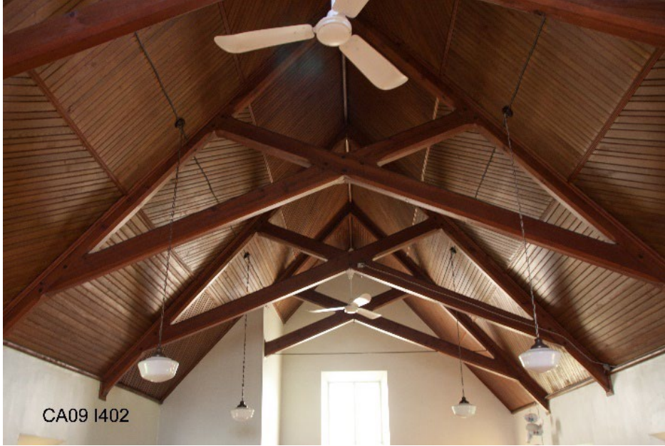
Wood ceiling with scissor truss detail. (Source: Anglican Archives, n.d.)
