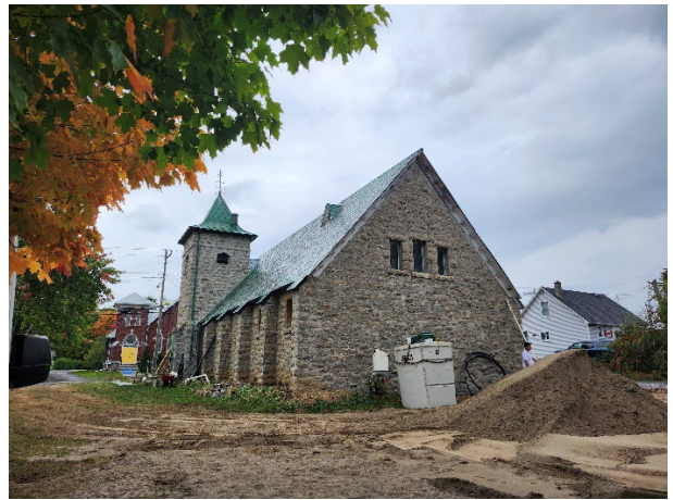
View of rear (east) elevation. Source: City of Ottawa, 2025.
