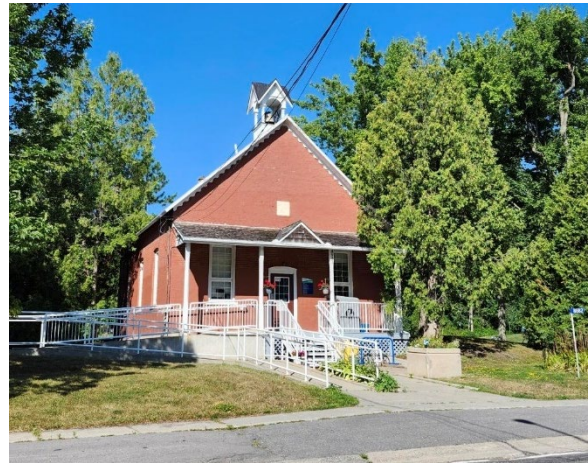
Former Vernon Schoolhouse at 8682 Bank Street. Source: City of Ottawa, 2025.
