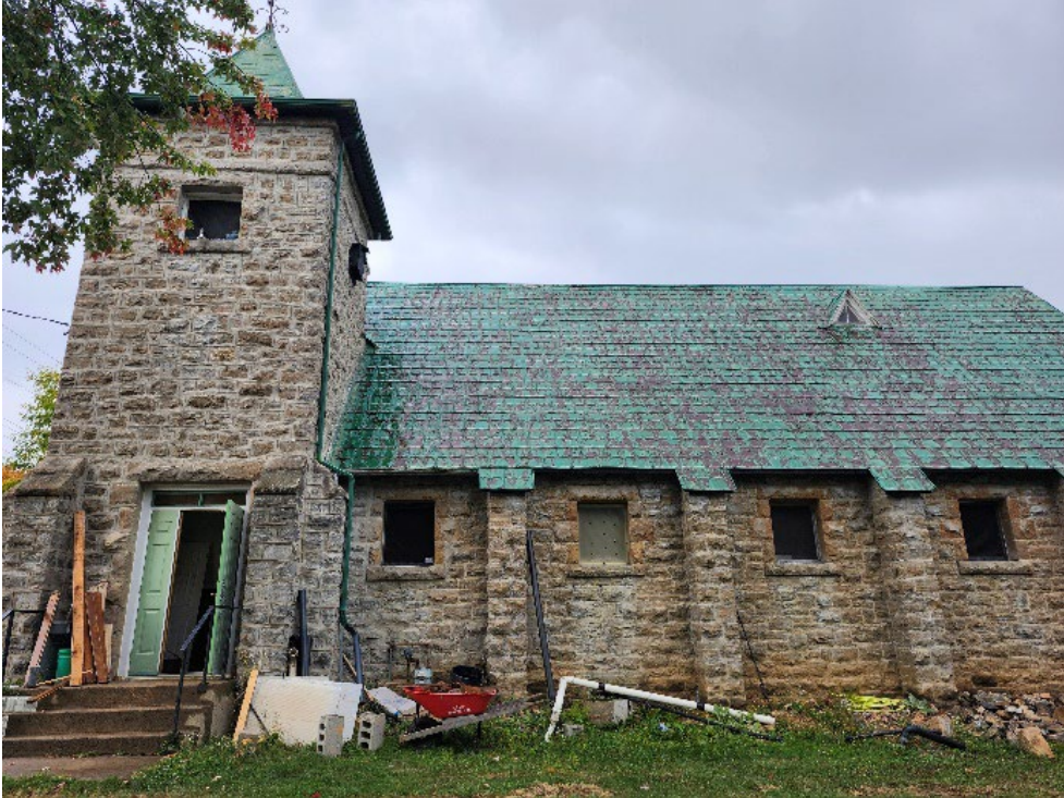
South elevation with main entrance through tower. (Source: City of Ottawa, 2025.)
