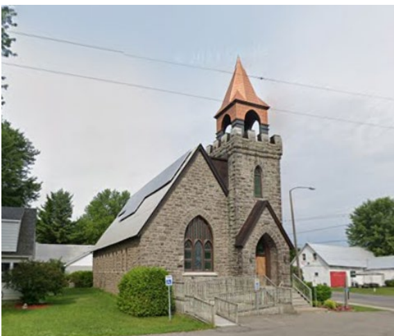
St. Mary's Anglican Church, 1171 Smith Road, Navan. Source: Google Street View, 2021.
