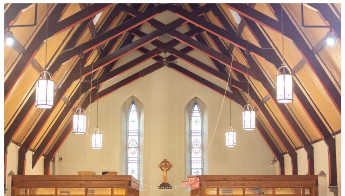
St. Albans Anglican Church, 454 King Edward Avenue. Source: https://stalbanschurch.ca/ .
