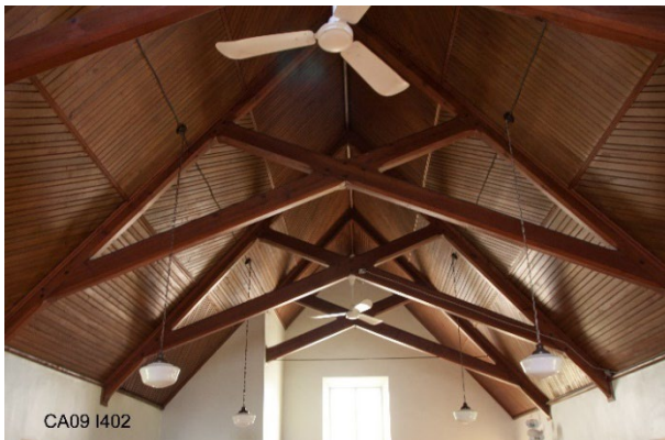
Timber ceiling with scissor trusses. Source: Anglican Archives.
