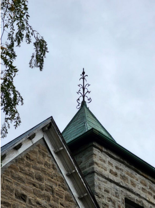
Tin pyramid roof and metal finial.
