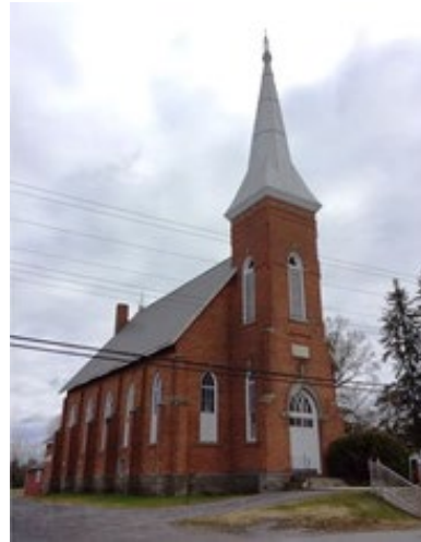
Osgoode Presbyterian Church. Source: City of Ottawa, 2025.
