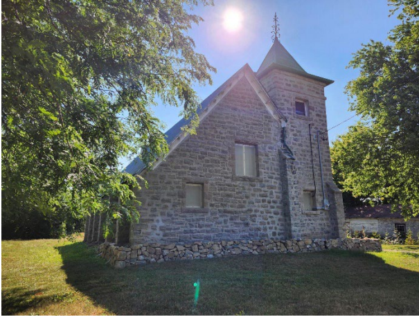
Front (west) façade facing Bank Street. Source: City of Ottawa, 2025.
