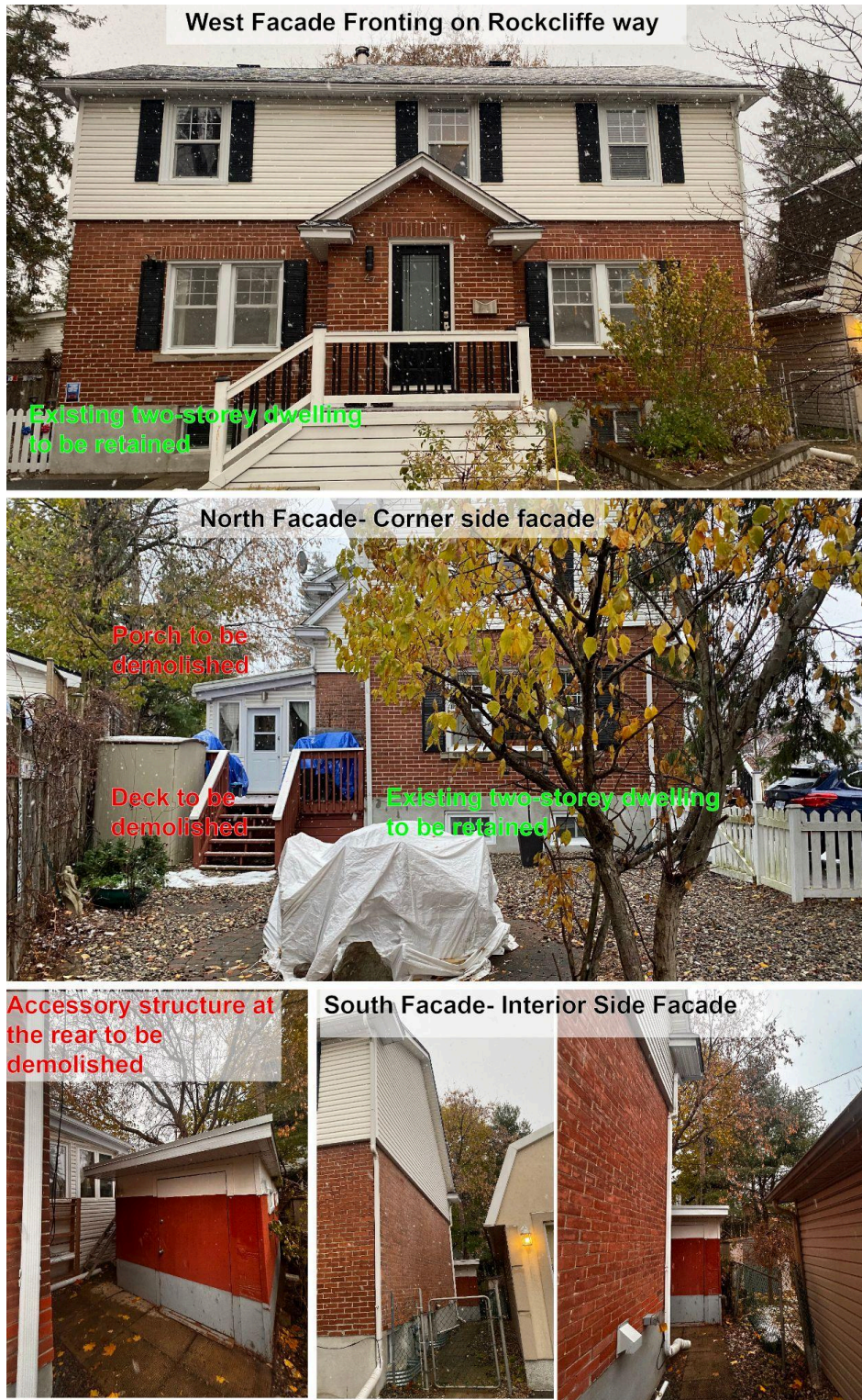
Fig 3. Subject property showing existing dwelling to be retained, and existing rear accessory structure deck and porch to be demolished.
