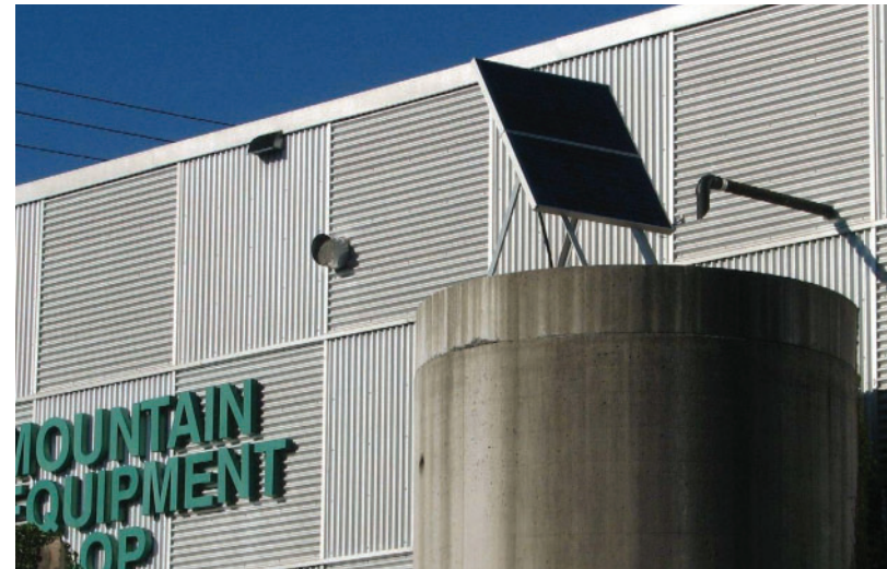
Figure 73: This commercial building collects solar energy and rainwater.
