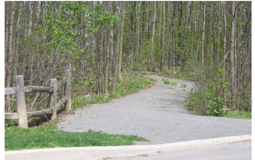
Figure 40: This trail is designed with limited amenities and a stone dust surface to reflect its more natural setting in a woodlot.
