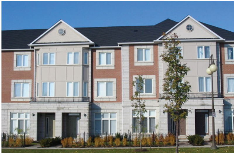
Figure 57: The ground floor treatment to doors and windows reinforces the pedestrian environment.
