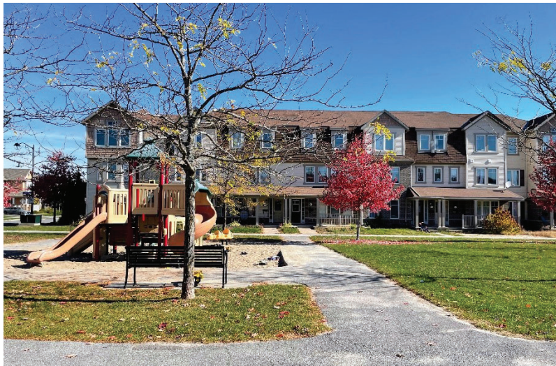
Figure 21: Rear garages enable dwellings to front directly onto a neighbourhood park, providing a greater sense of spatial enclosure in the park and natural surveillance opportunities.
