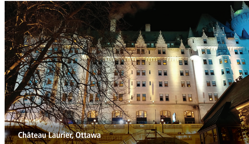
Figure 36: The temporary exterior lighting set up for the 2017 Crushed Ice World Championship highlights the architectural characteristics of the historic building.
