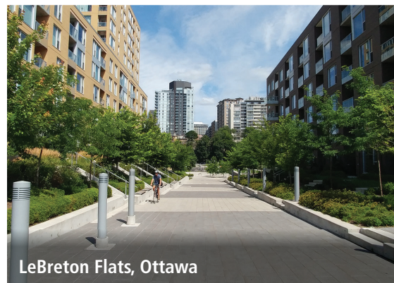
Figure 49: A mid-block connection in a residential area that provides convenient access for pedestrians and cyclists.
