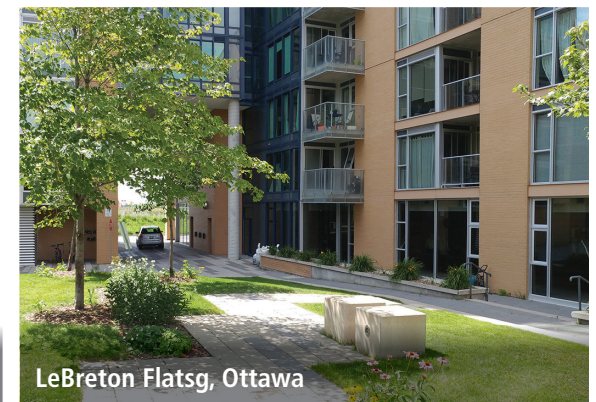
Figure 47: A residential courtyard offers a quasi-public amenity area.
