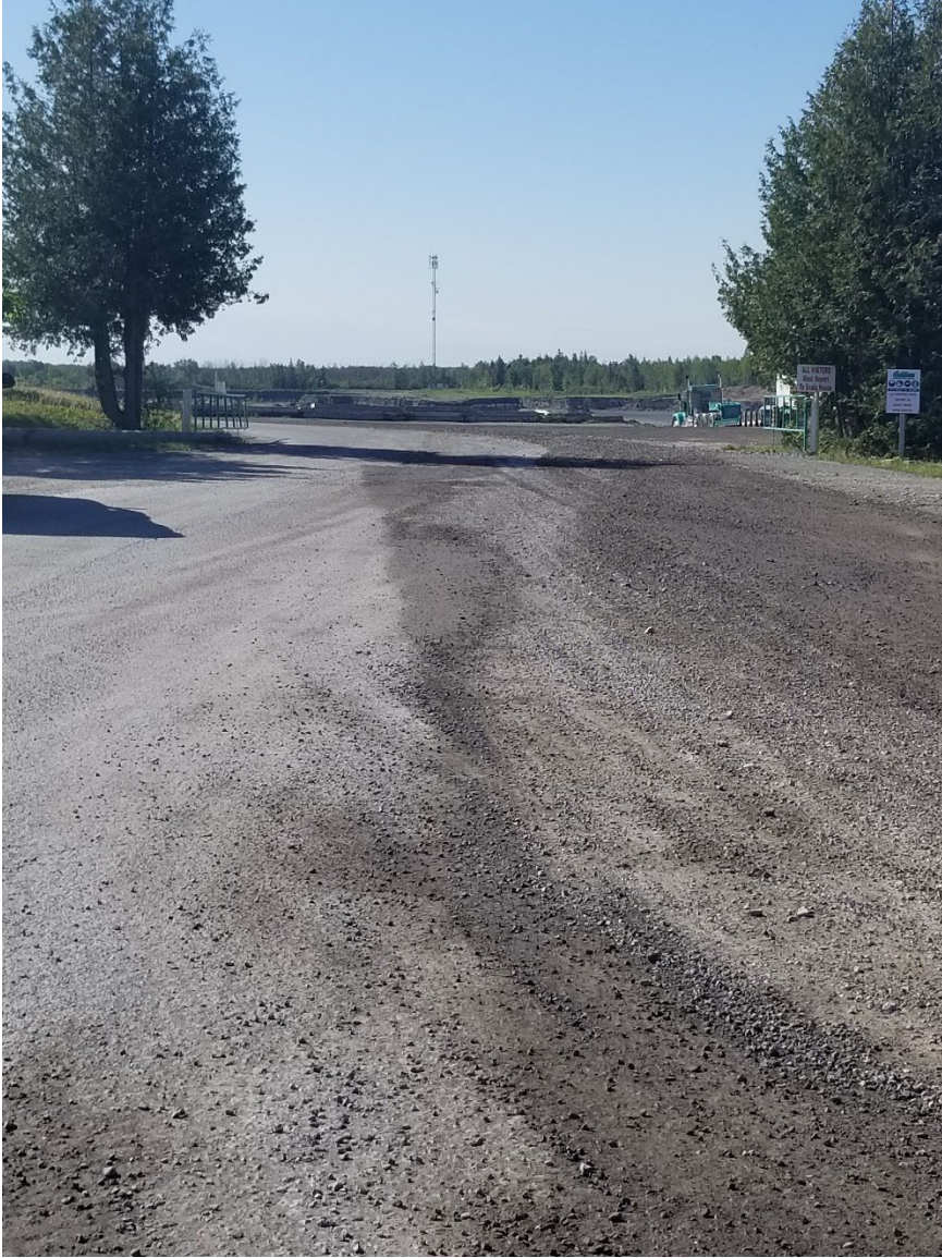
Goulbourn Quarry entrance off Flewellyn Rd. May 31, 2021 G McLaren
