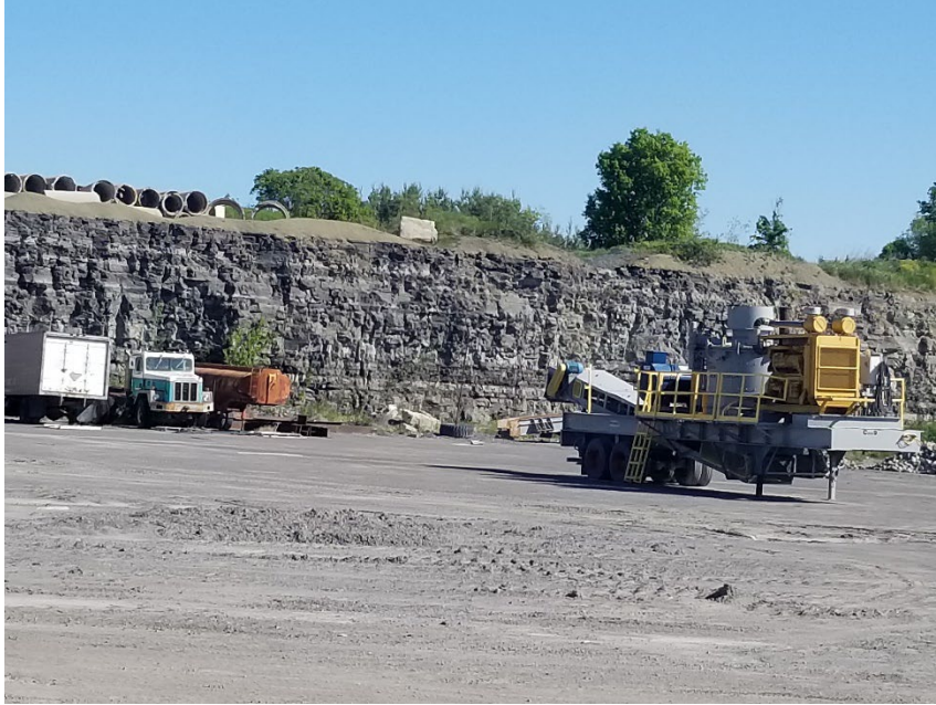
Goulbourn Quarry north quarry face at extraction limit 200 metres from Flewellyn Rd. May 31, 2021 G McLaren
