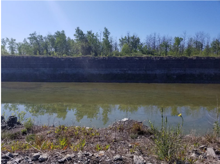
Looking at west face, quarry 2 nd lift, toward Munster Rd. Area depleted of marketable stone. May 31, 2021 G McLaren
