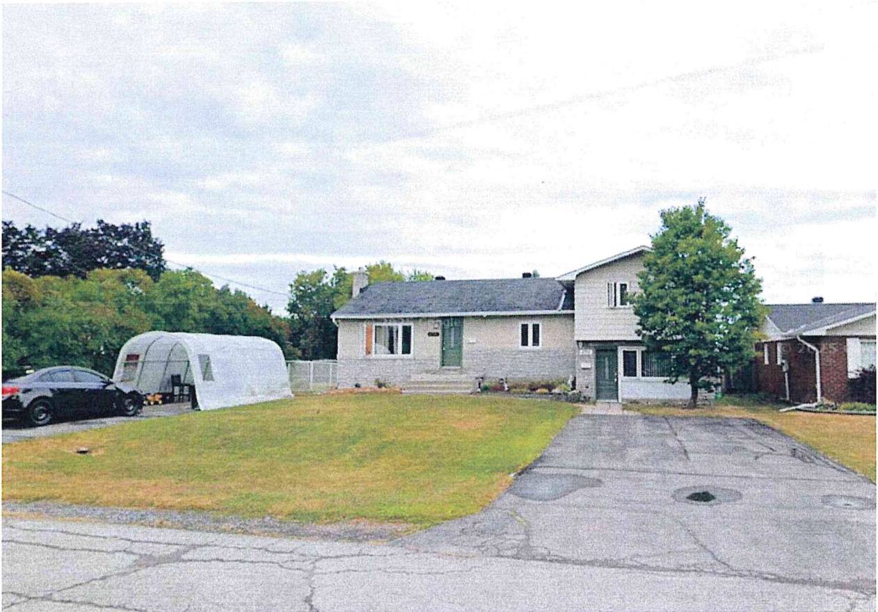
Figure 6 – Front Facing Semi Detached immediately to the east of 6719 Barsona Place.
