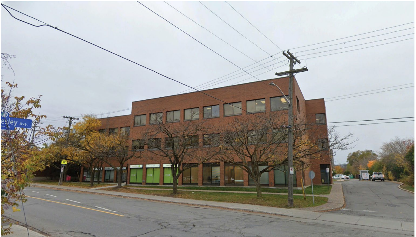
Figure 4: Street view image of the subject property's frontage on Broadview Avenue.
