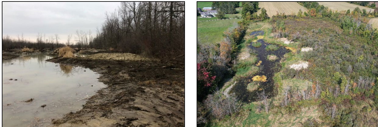
Figure 2: Wetland restoration project completed near North Gower in Rideau-Jock ward
