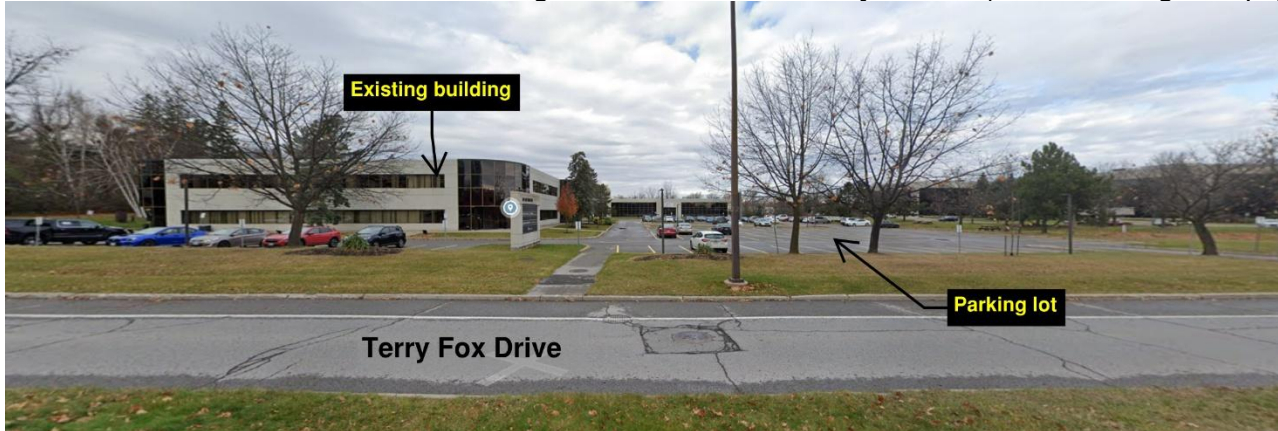
Figure 3: Streetview of Subject Site. (Source: Google Maps).
