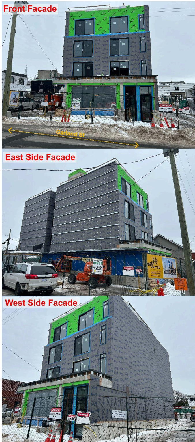
Fig.5. Subject property showing the building under construction.
