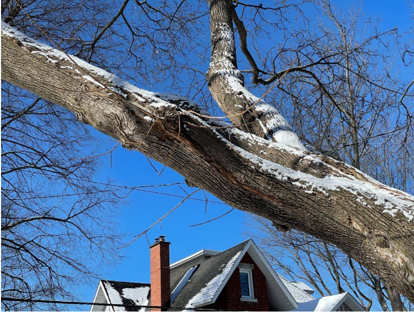
Photo 2: Tree 1, horizontal crack large branch hanging over road
