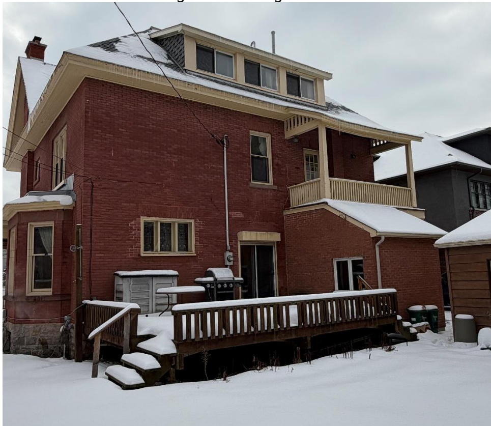
Figure 7: Existing Rear Yard Condition of Detached Dwelling
