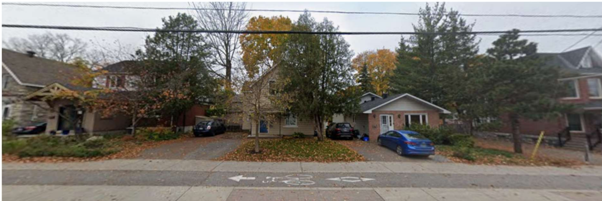
View across the street. It is likely that a number of properties will be redeveloped along Churchill when the new Bylaw comes into effect, given that the new bylaw will likely allow 0 minimum setback to the front lot line.
