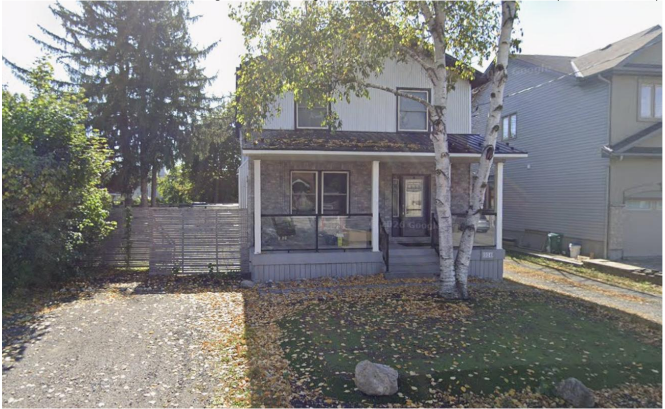
Figure 3: Existing Building at 324 Duncairn Avenue (to be retained)
