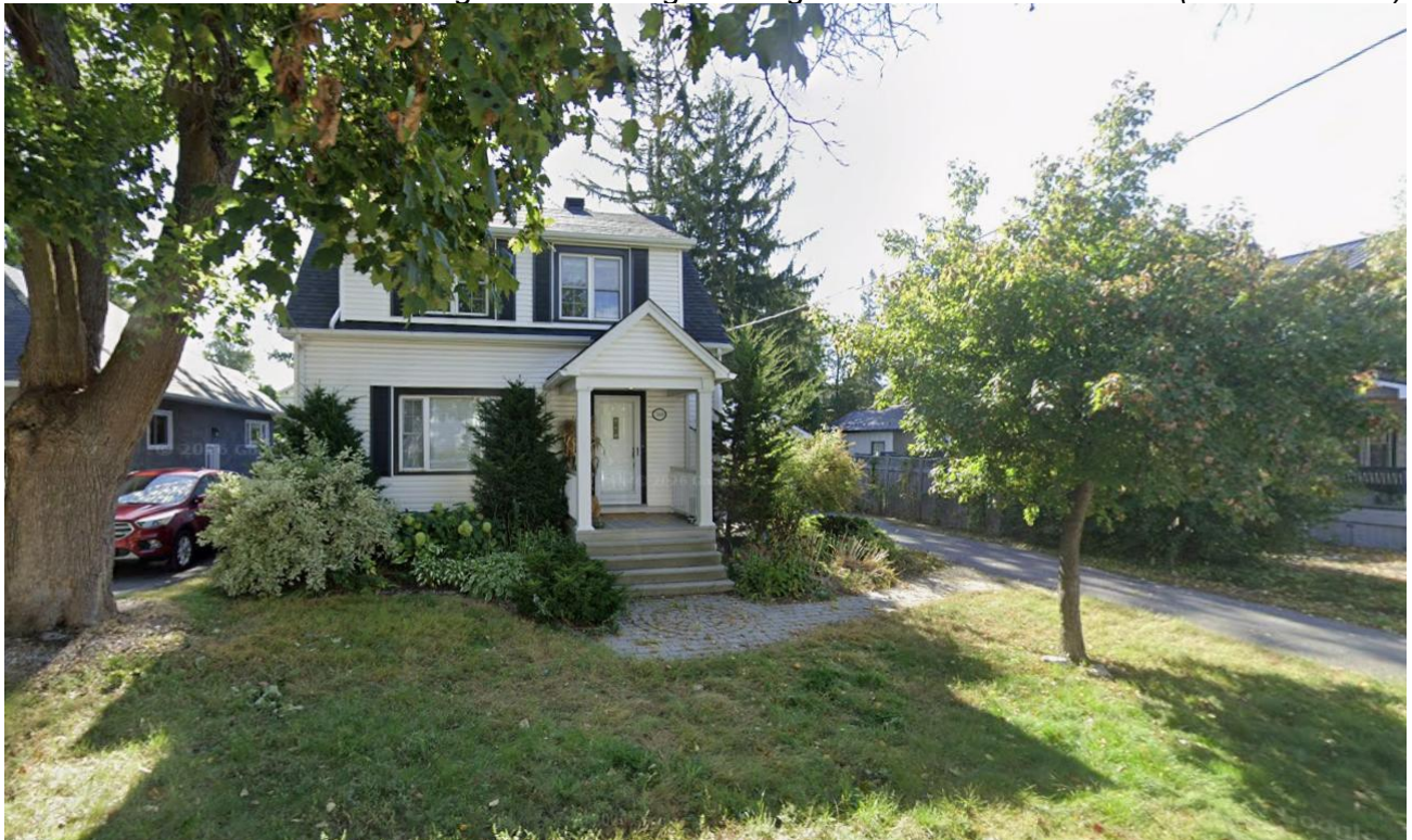
Figure 4: Existing Building at 318 Duncairn Avenue (to be retained)
