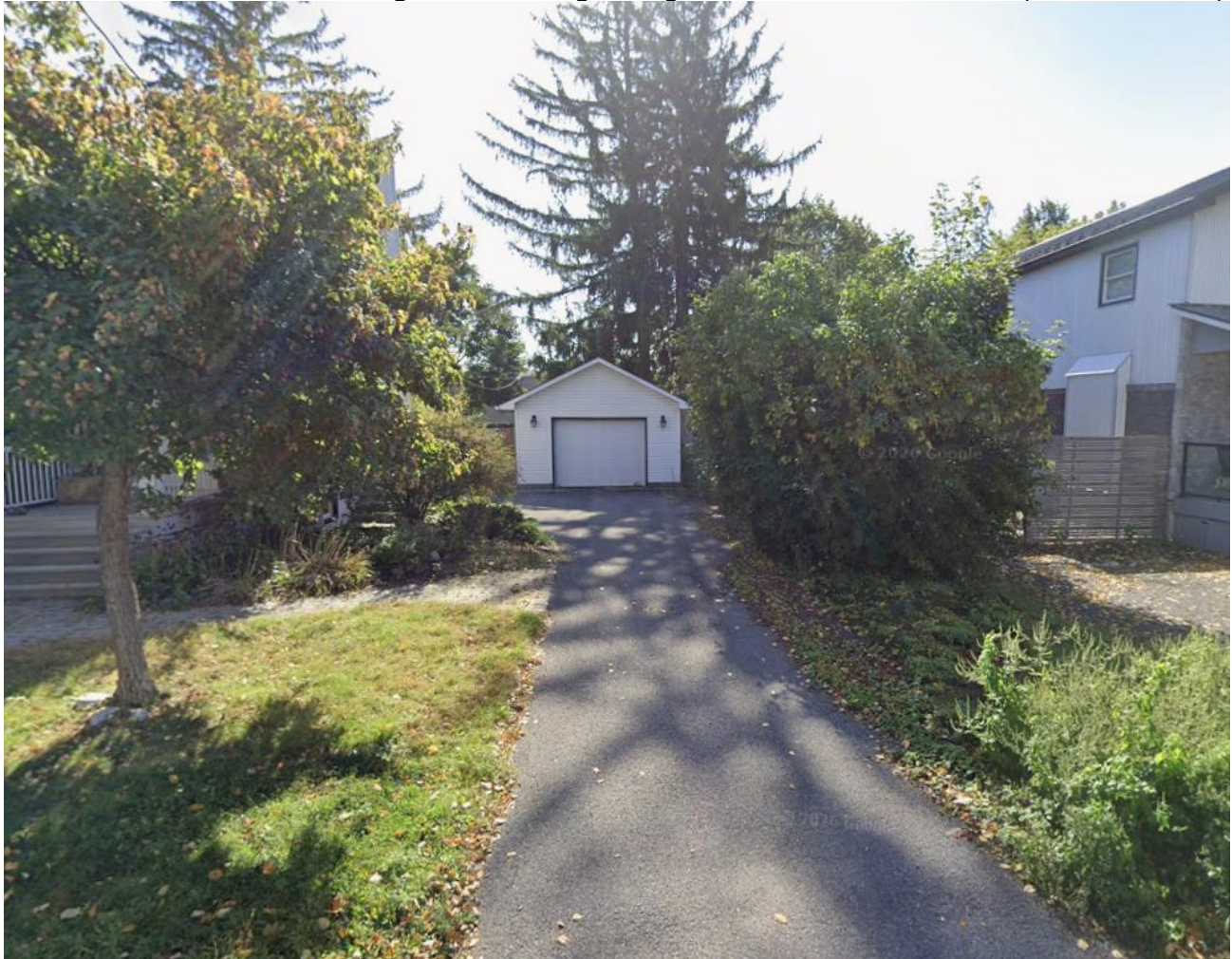
Figure 5: Existing Garage at 318 Duncairn Avenue (to be removed)
