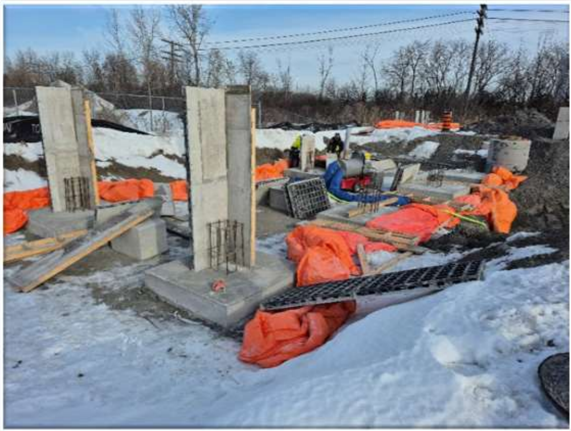
Electrical equipment foundation
