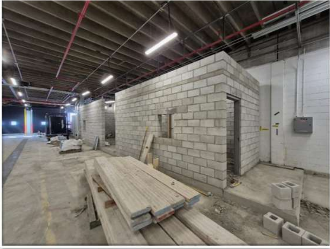
Electrical room construction
