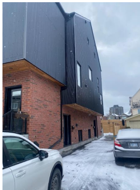
Figure 3. Image of the cantilevered roof
