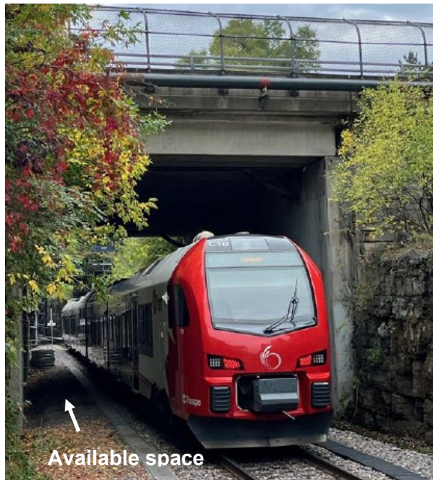
Figure 5: O-Train Line under Carling Avenue Bridge Showing Available Space
