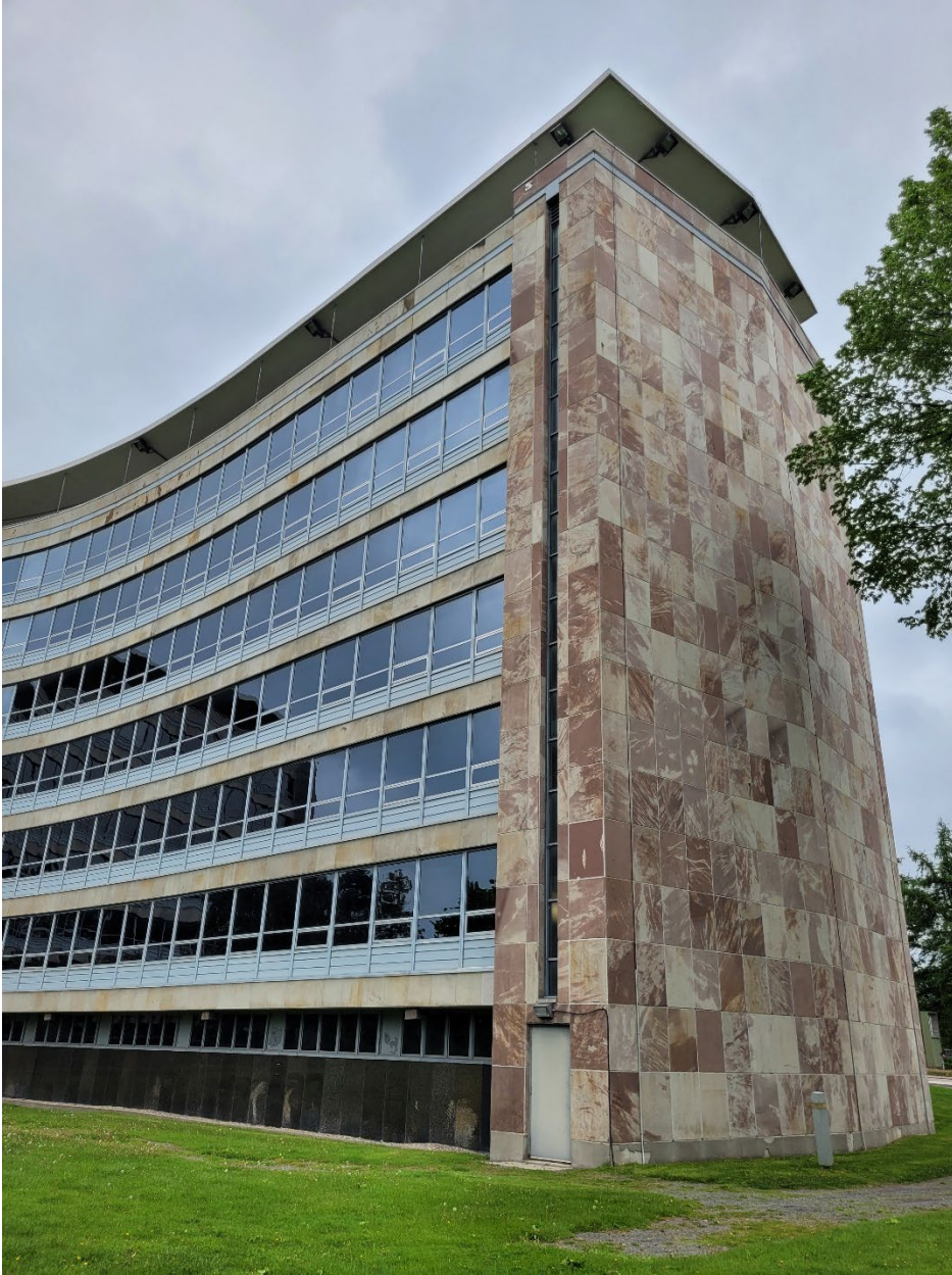
Image showing the sandstone cladding on the north wing wall.
