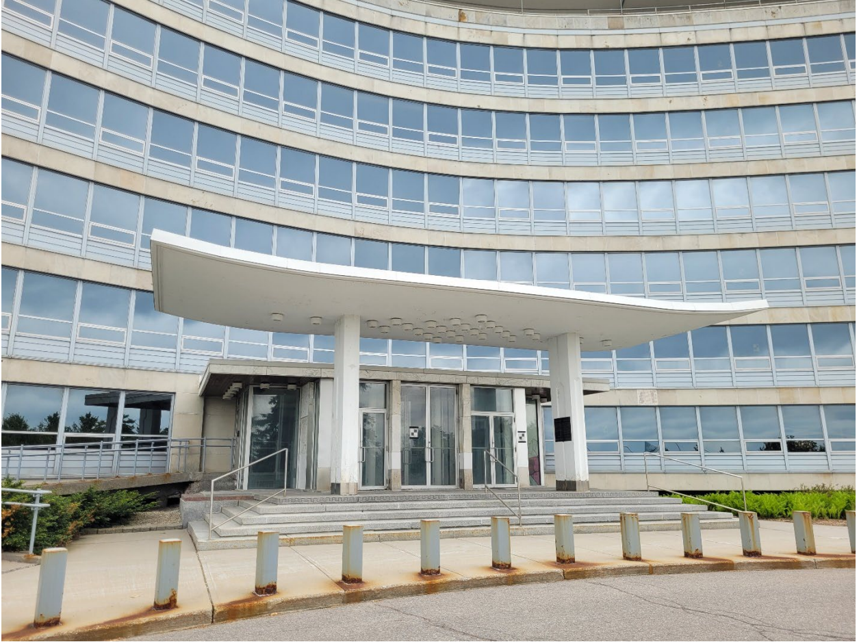
Image showing the flared entrance pavilion with glazed curtain wall behind.
