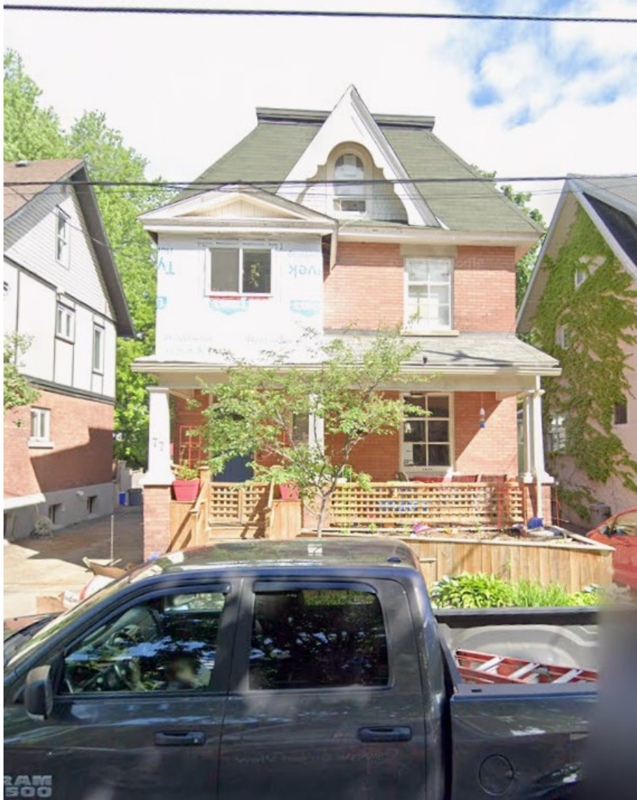
Figure 3 – view of the subject property from Glen Avenue
