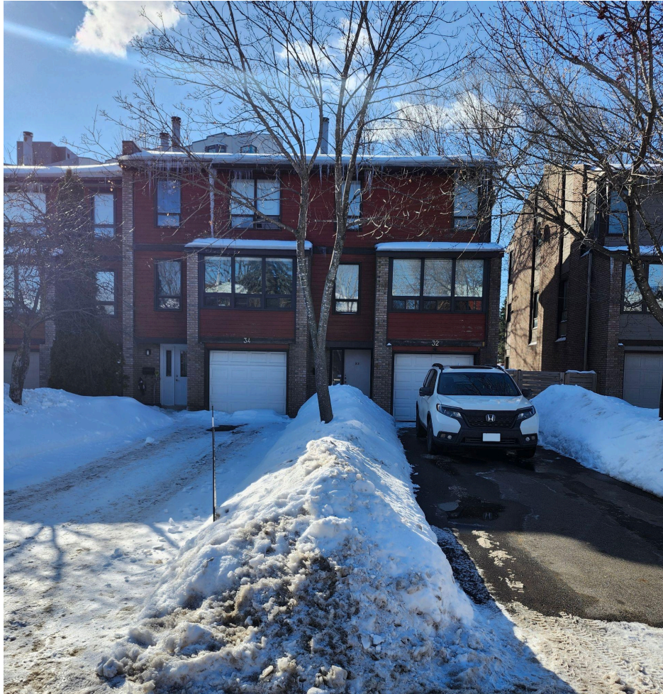
Figure 7: Current photo of the property (Feb 2026)
