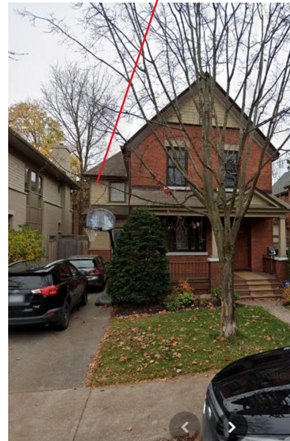
House at No. 24, with existing addition with 1.2m Side Yard.
