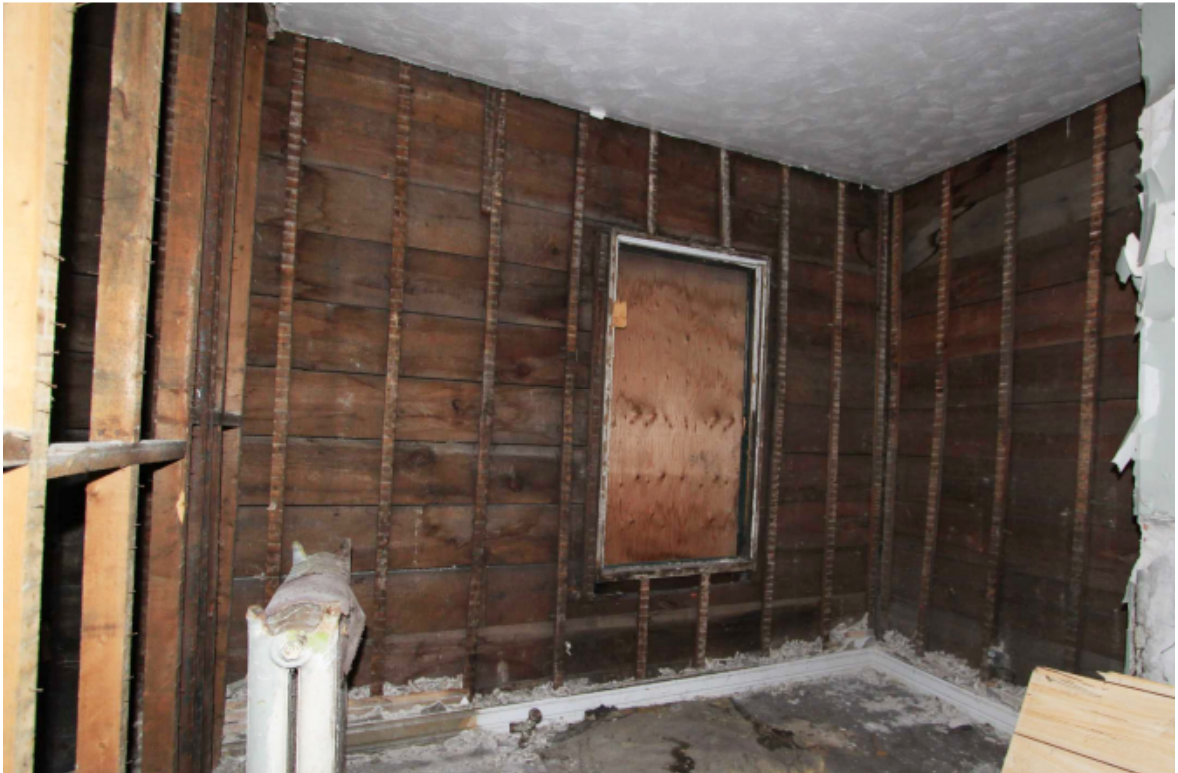
Figure 6. Plank Framing System
