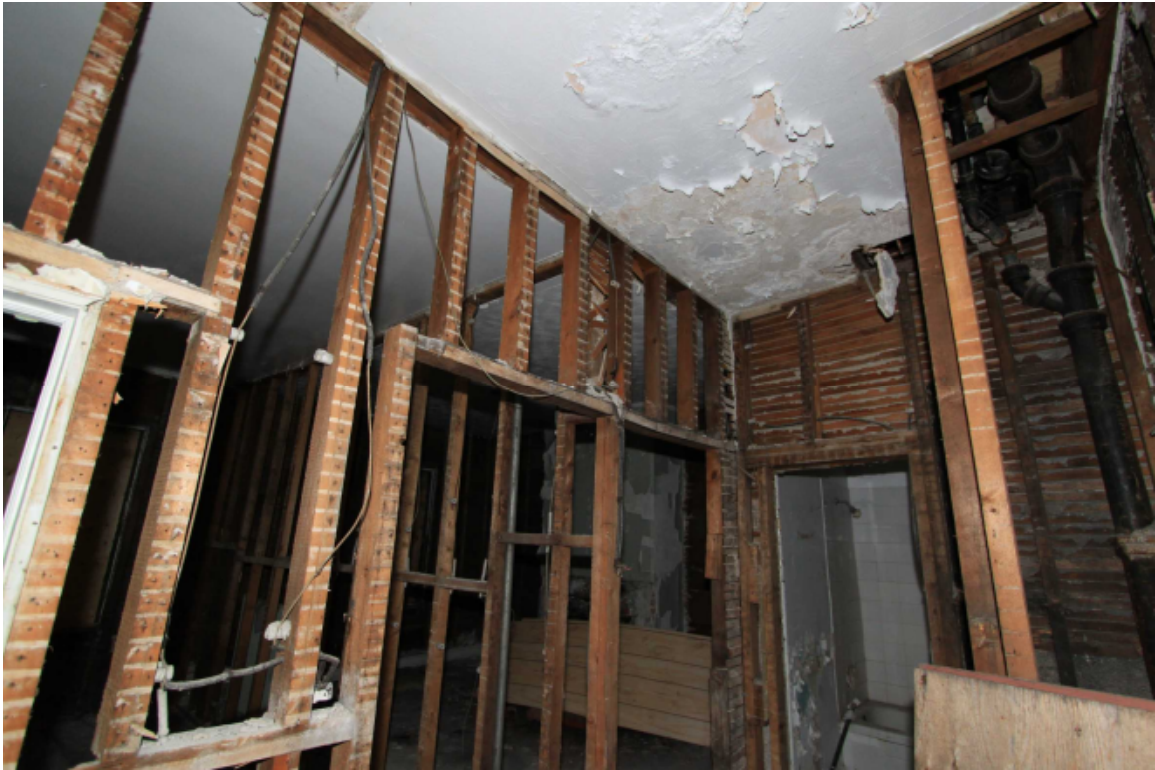
Figure 9. Interior Partition/Loadbearing Walls
