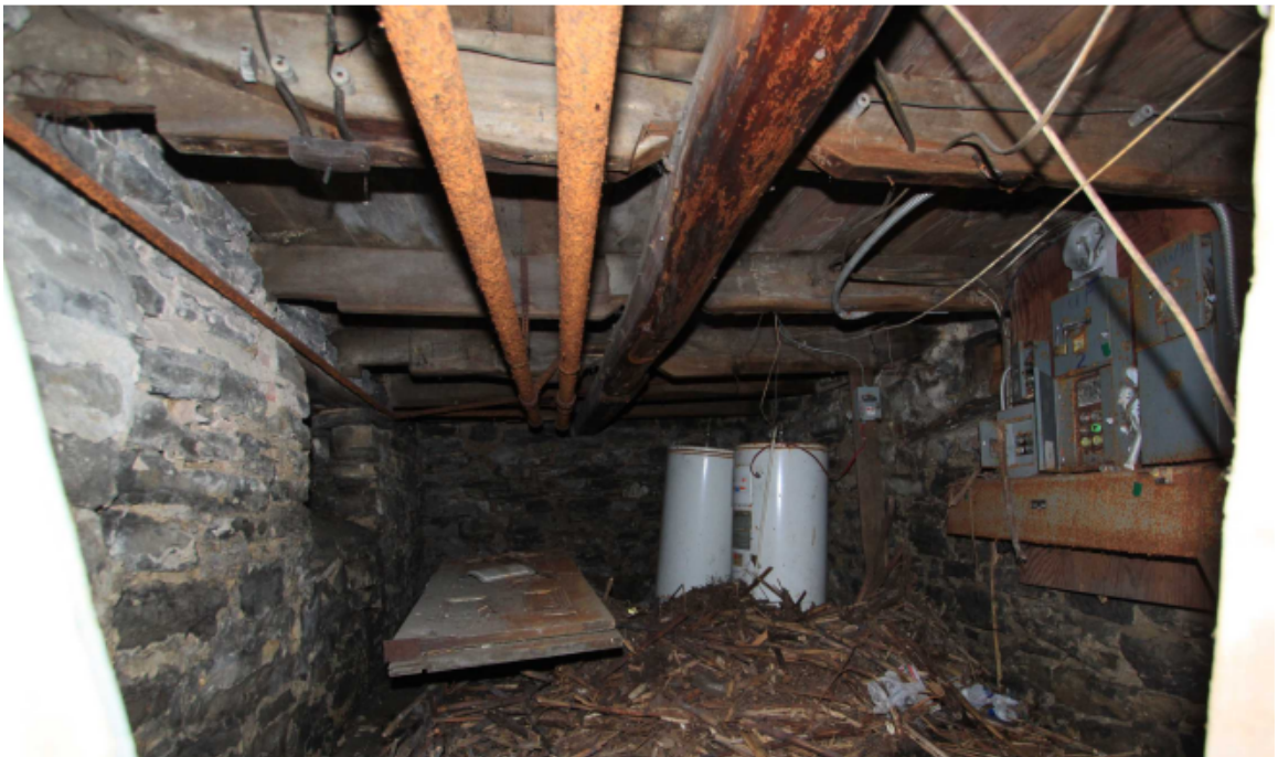
Figure 5. Ground Floor Joists
