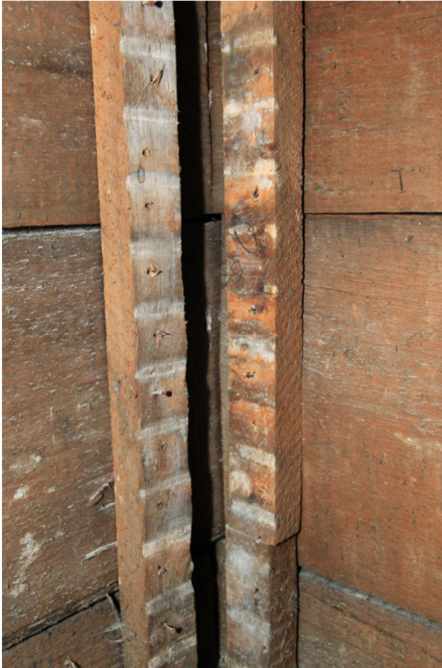
Figure 7. Planks are Overlapped in Corners
