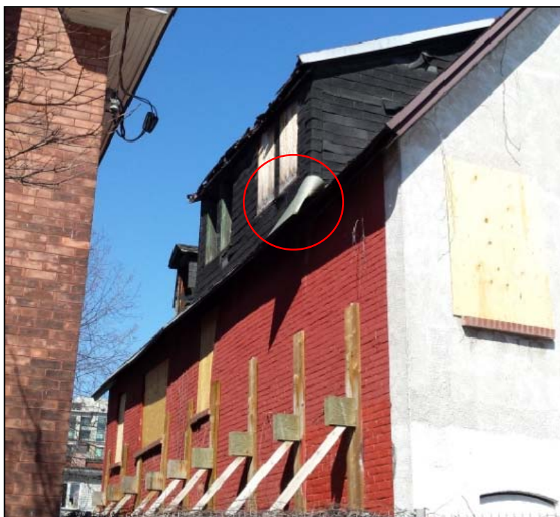
Image 1: 197 Wilbrod St. Sheet Metal Cladding on West Roof
