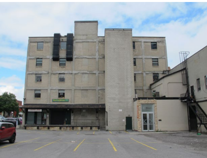
South elevation and south wing
