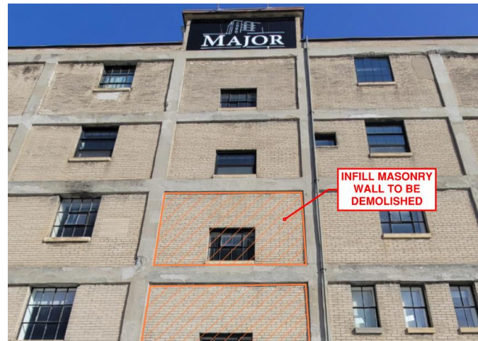
Figure 1 - Western facade with infill masonry
