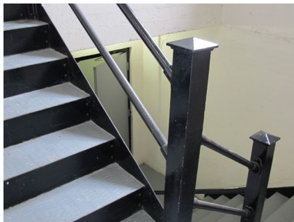
Typical interior stair
