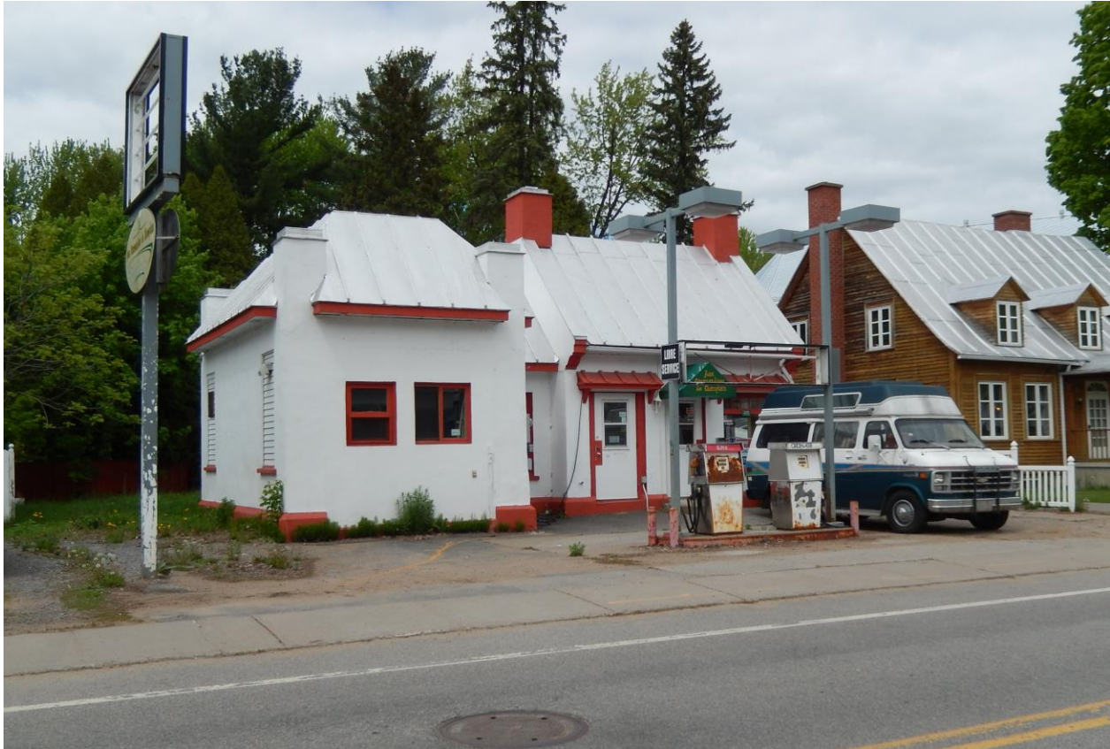
Figure 14: Built in 1935 in Champlain Quebec; the Champlain Oil Company Service Station with its distinct cottage form located at 975 Rue Notre Dame, is a designated historic site. The garage door on the left has been closed in.
