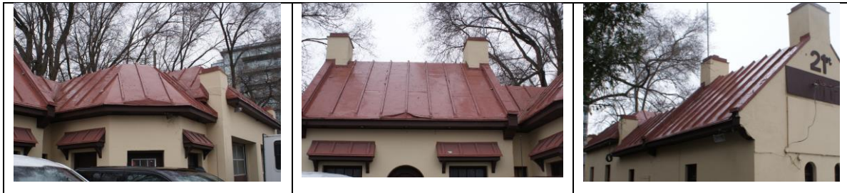
Figure 3A: images of the Roof
