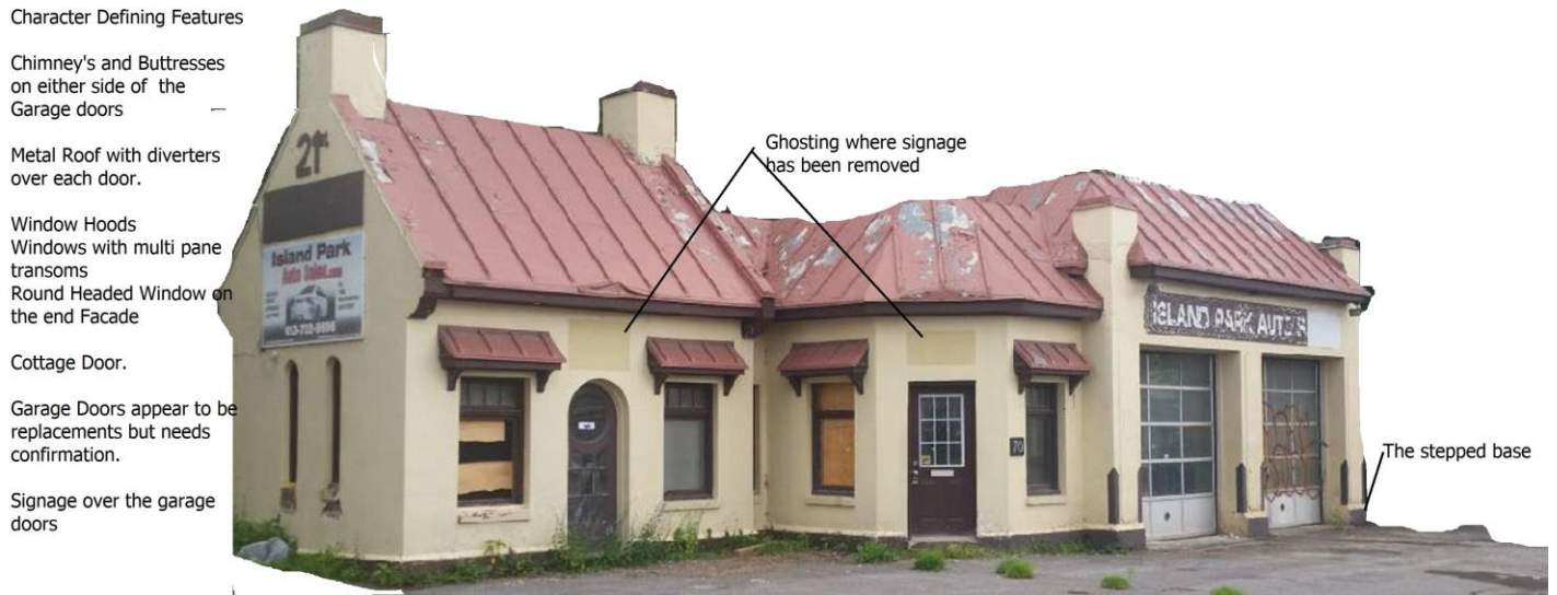
Figure 4: Annotated view of the Service Station highlighting the identified attributes. Source: Commonwealth
