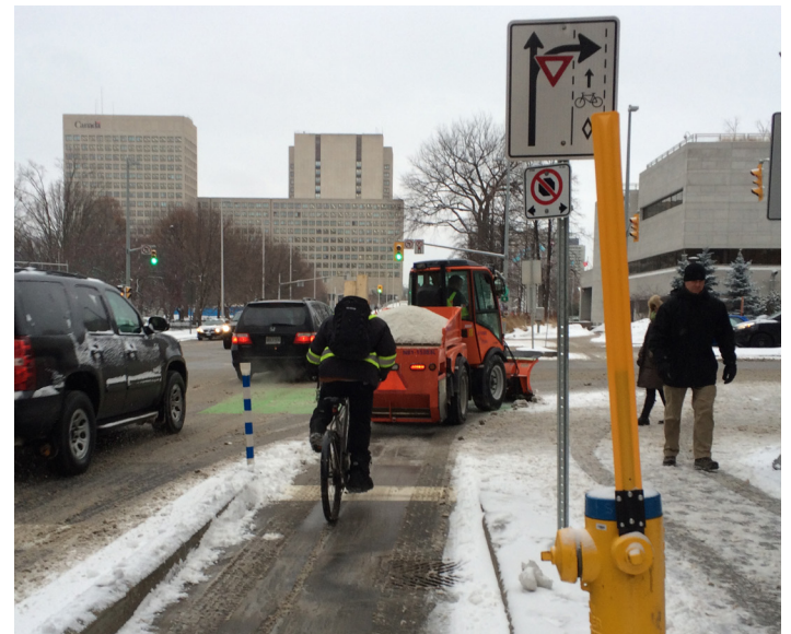
Image 6.6. Ottawa's snow plow clearing Laurier Avenue bikeway with reflective post on features
