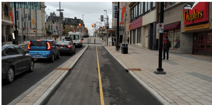
Image 6.4. Side inlet catch basins at Rideau Street
