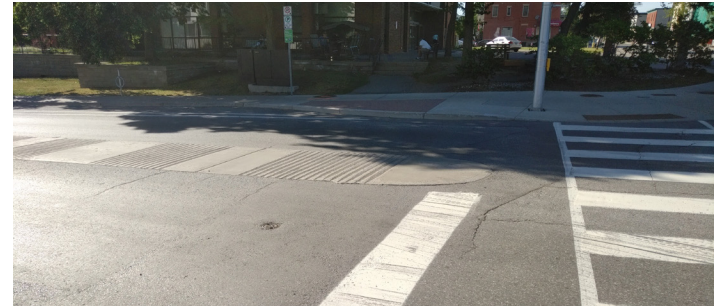
Image 5.4. Example of flush concrete ribbed centreline hardening at Gladstone Avenue and Rochester Street
