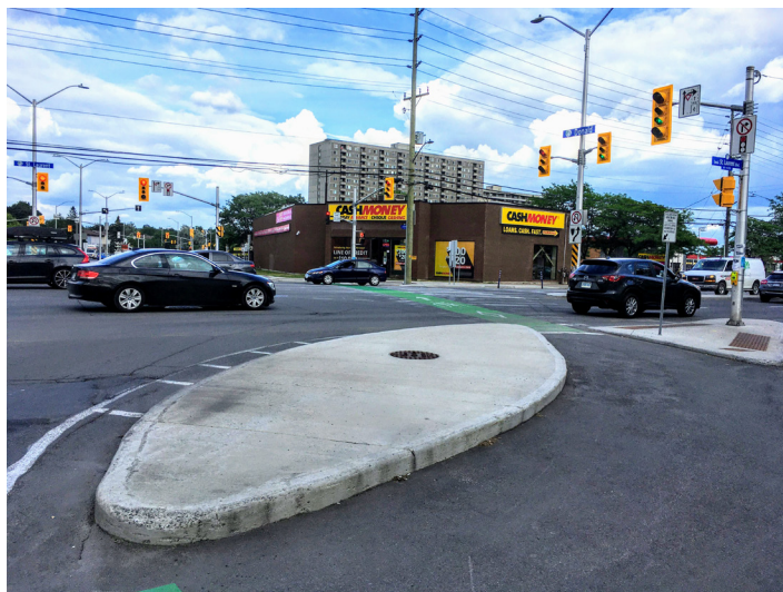
Image 5.5. Example of corner safety island at Donald Street and St-Laurent Boulevard
