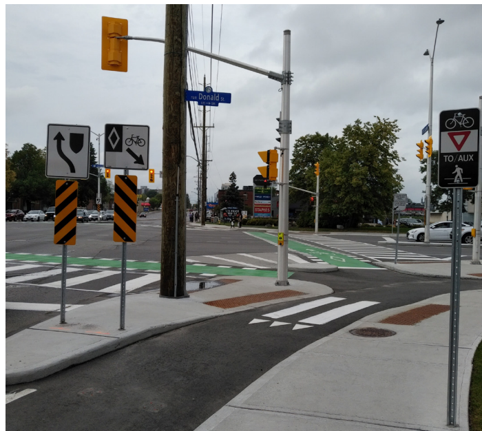
Image 6.7. Raised corner safety island and raised features in standard protected corner at Donald Street and St. Laurent Boulevard
