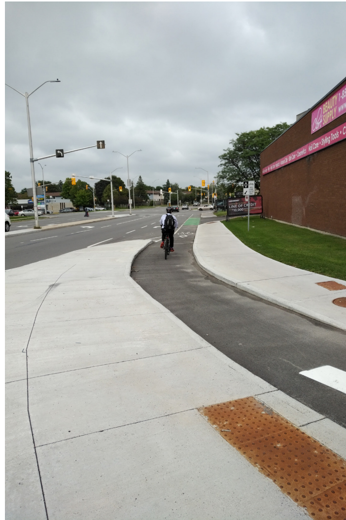
Image 5.9. Example of transition from cycle track to on-street bike lane at Donald Street and St-Laurent Boulevard
