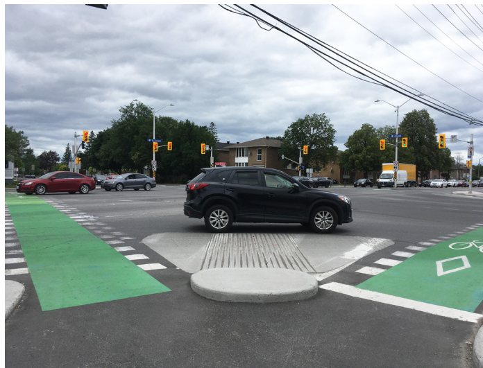
Image 6.10. Flush concrete grooved apron at Donald Street and St-Laurent Boulevard
