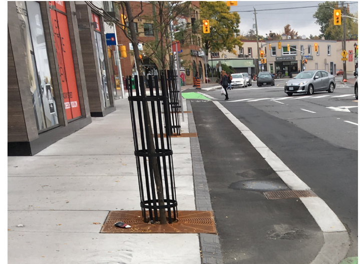
Image 5.1. 3.0 m sidewalk on Beechwood Avenue
