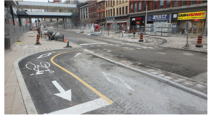
Image 6.1. Half-height curb between sidewalk and cycle track on Rideau Street
