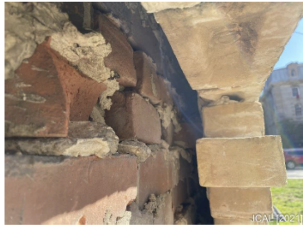
Photo 1d: Facing Brick and Cavity [JCAL (2021)]
