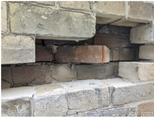
Photo 1g: Cavity and Diagonal Tying Brick [JCAL (2021)]
