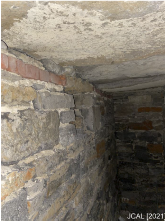
Photo 1e: Foundation and Stone Slabs [JCAL (2021)]
