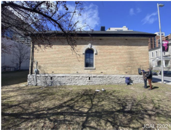
Photo 1c: South Elevation [JCAL (2021)]
