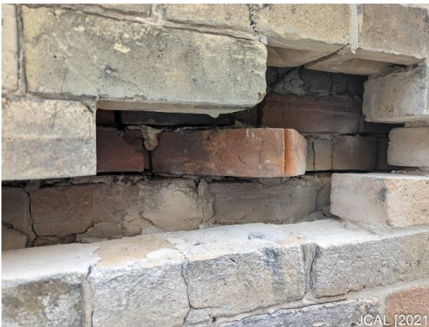
Photo 1g: Cavity and Diagonal Tying Brick [JCAL (2021)]
