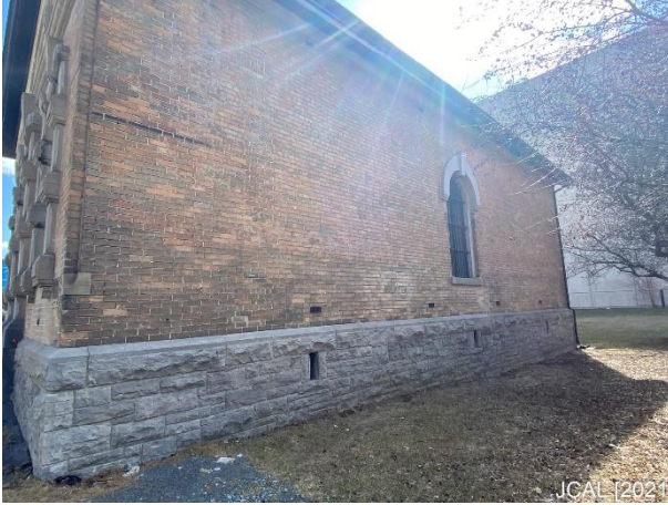
Photo 1a: North Elevation [JCAL (2021)]
