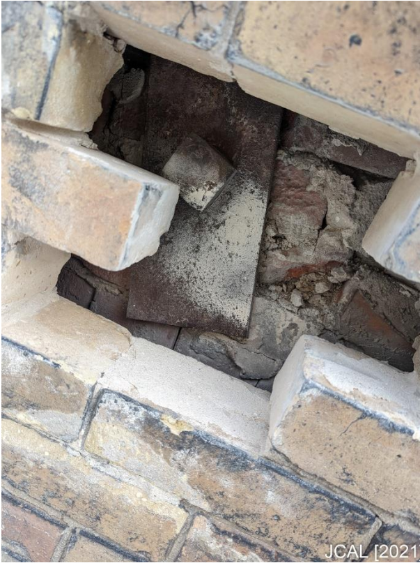
Photo 1i: Tie Rod End Plate [JCAL (2022)]
