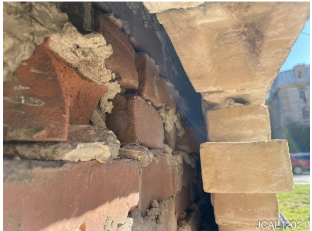
Photo 1d: Facing Brick and Cavity [JCAL (2021)]
