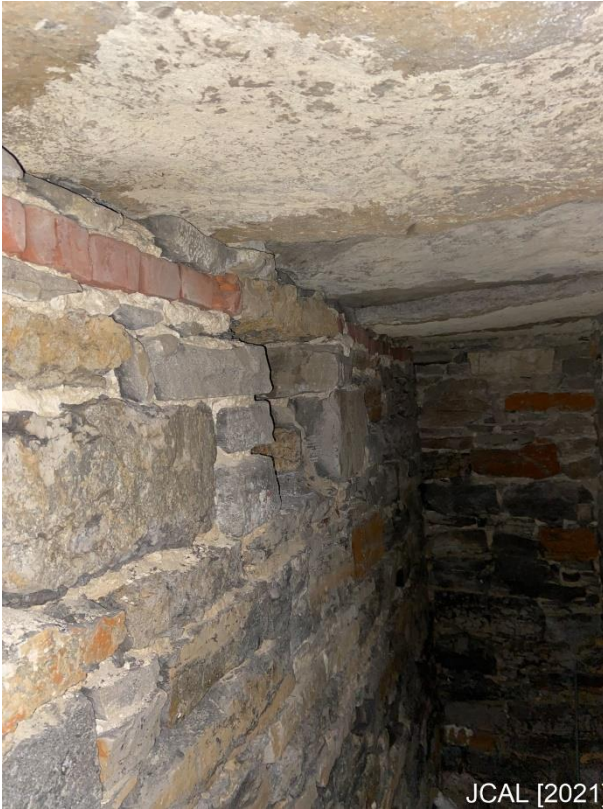
Photo 1e: Foundation and Stone Slabs [JCAL (2021)]
