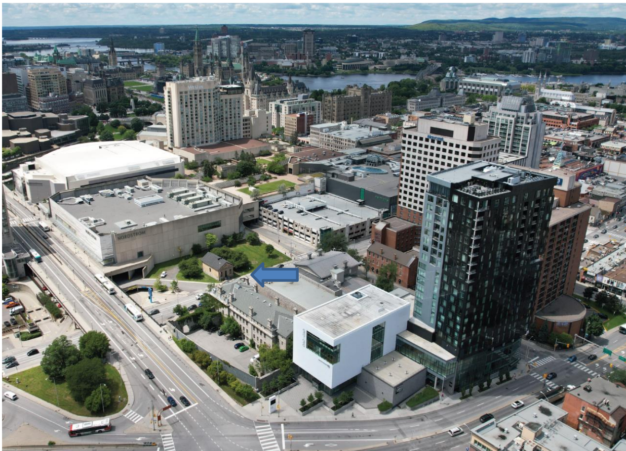
Figure 3: Bird's eye view illustrating the built context surrounding the development site (Site arrowed). Source: Zeidler, 2021.
