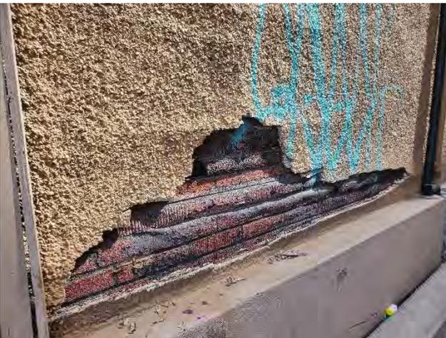
Figure 14B. Lower north corner of the west façade showing previous cladding, asphalt shingle-like material.
