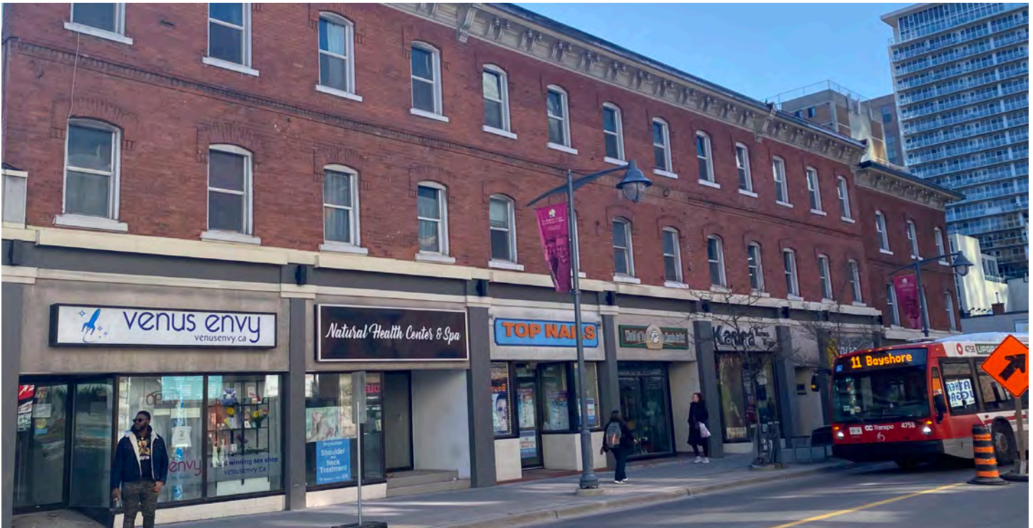
Figure 17: Commercial flat roofed building on Bank Street with ground floor retail.
