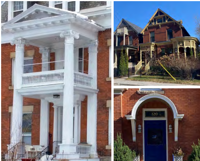
Figure 15: Examples of the HCDs' porch types, balconies and canopies.
