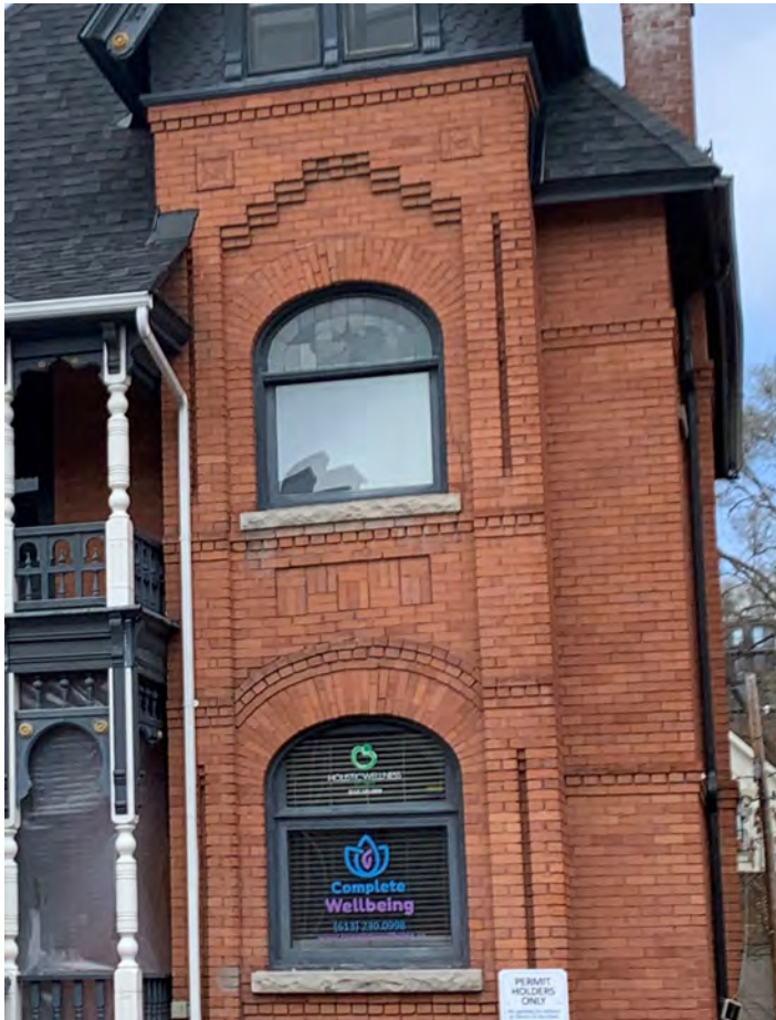
Figure 13: An example of Centretown's historic brick at 355 Waverley Street, including detailed string courses and voussoirs.
