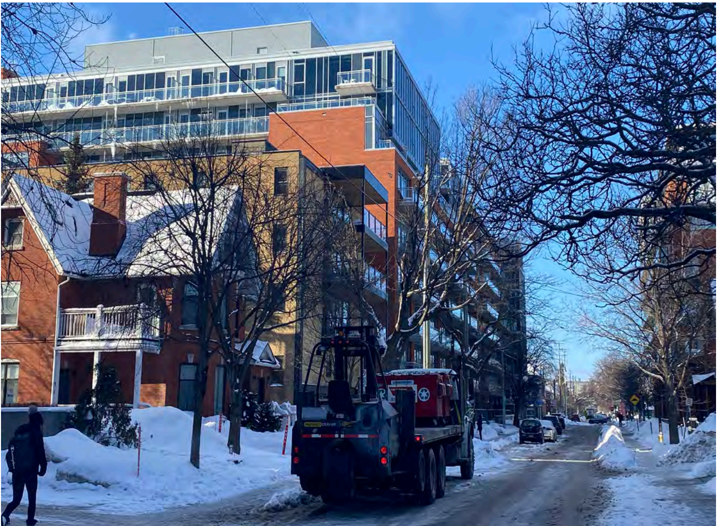
Figure 26: Image of a new construction on McLeod Street, with stepped back upper floors that provide massing relief and transition down to the lower scale properties in the middle of the block.
