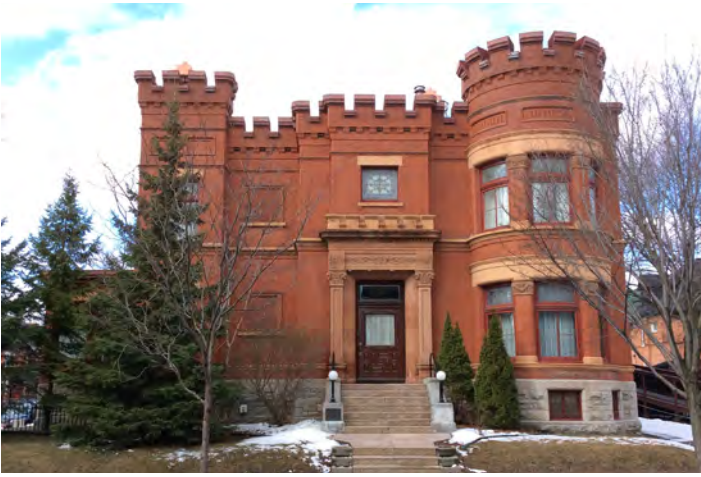
Figure 11: Historic Birkett House Credit: ERA Architects Inc
