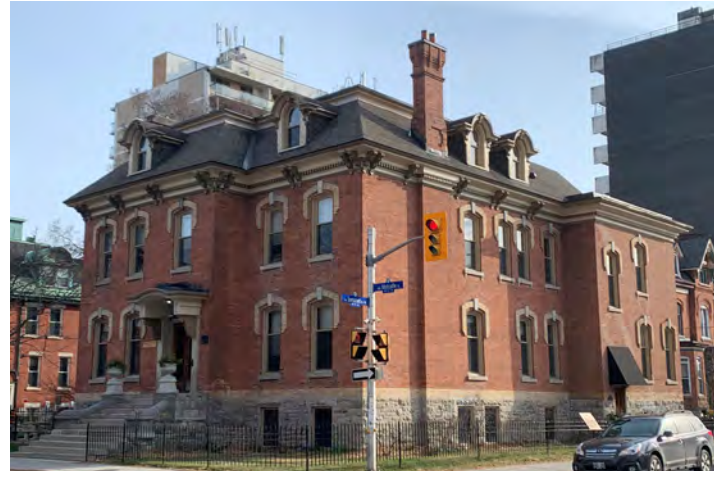
Figure 12: Campbell House with a variety of roof elements and dormers. Credit: ERA Architects Inc
