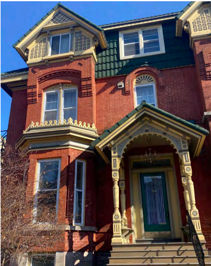
Figure 16: Examples of intricate wood work in the gable, brackets, corbeling detailed brick work, as well as iron cresting.
