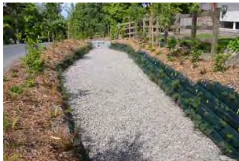
Figure 10: Roadside Ditch Enhancement Granular bottom and Vegetated Wall Side Slops
