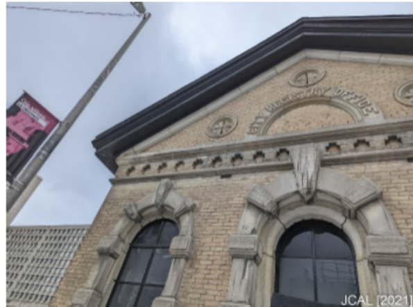
Photo 1b: Partial East Elevation [JCAL (2021)]
