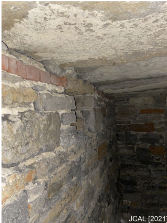
Photo 1e: Foundation and Stone Slabs [JCAL (2021)]
