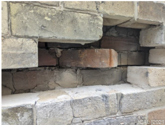
Photo 1g: Cavity and Diagonal Tying Brick [JCAL (2021)]
