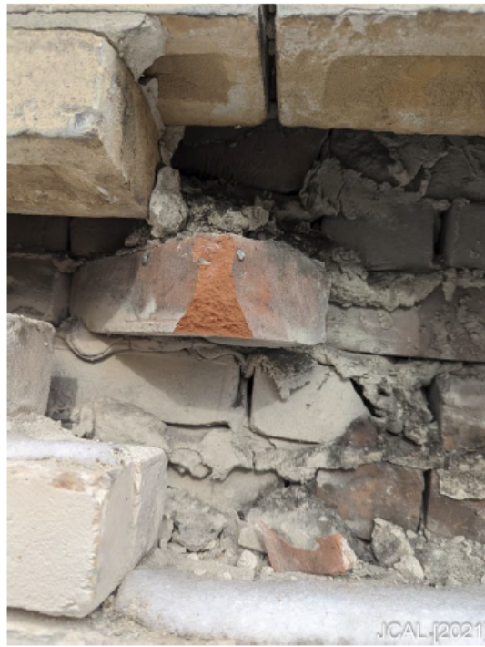
Photo 1f: Cavity and Diagonal Tying Brick [JCAL (2021)]
