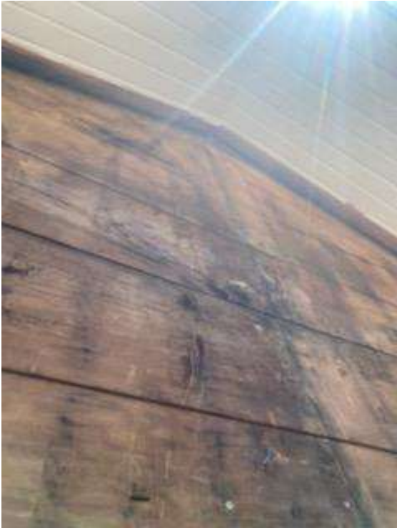
Fig. 6 and Fig. 7: Exposed boards after stucco panels were removed
