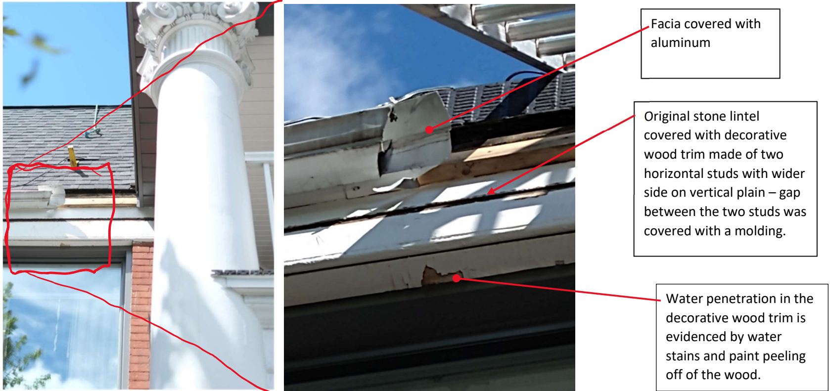
Fig. 8 and Fig. 9: Front of house – upper fascia and decorative trim above 2 nd floor windows: Photo shows that fascia was covered with aluminum. Rain gutter was also installed. Water penetration is evident. Long term concern is water damaged wood will attract infestation of insects such as carpenter ants.
