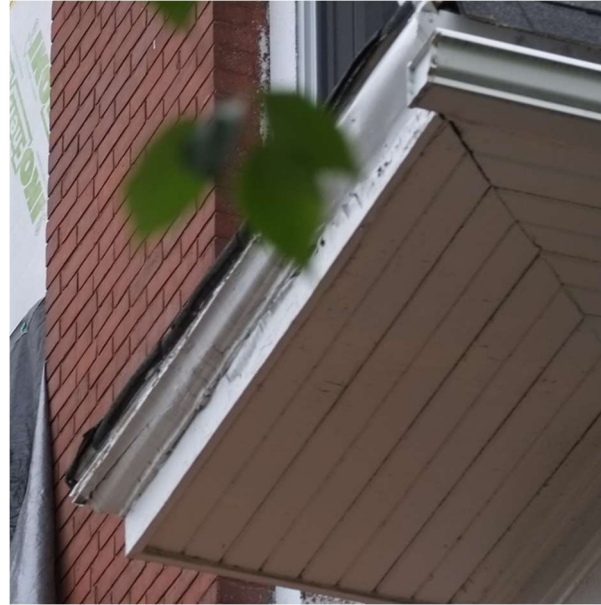
Fig. 10 and Fig. 11: Crown mouldings have deteriorated pass point of repair. Aluminum caps on the end of the crown mouldings are visible in both photos
