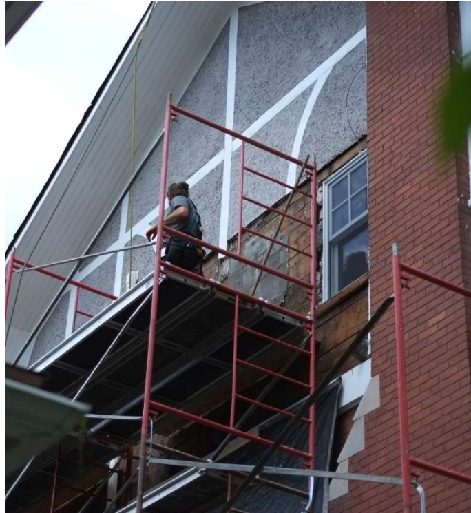
Fig. 6 and Fig. 7: Exposed boards after stucco panels were removed
