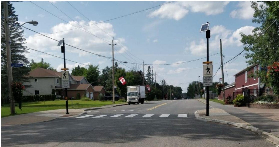
Figure 5 – Image of Type C PXO Located on Carp Road in the Village of Carp
