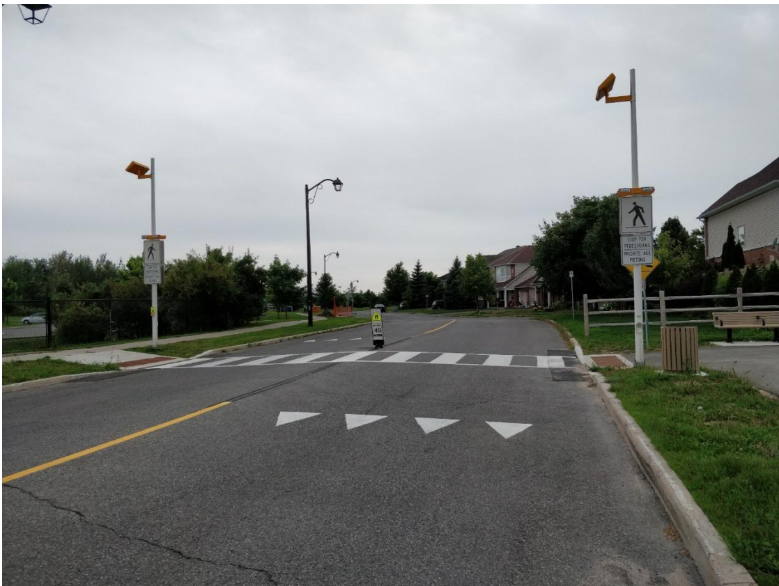
Figure 6 – Image of Type C PXO Located at Aquaview Drive and the Trillium Pathway
