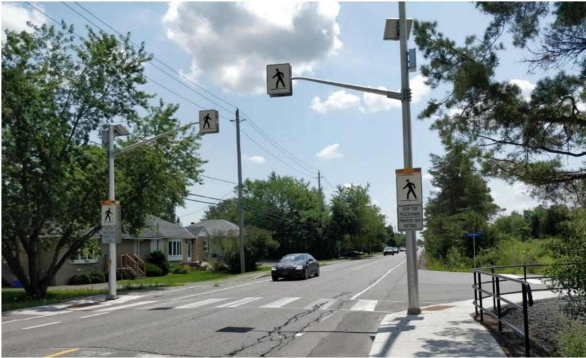
Figure 3 – Image of Type B PXO Located at Blair Road at Appleford Street
