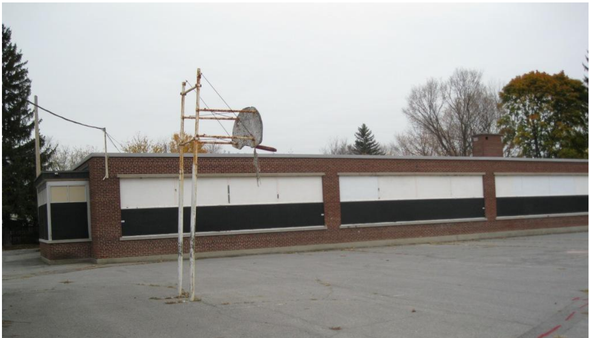
1949 Annex to be demolished, replaced with new structure to be linked to heritage building.
