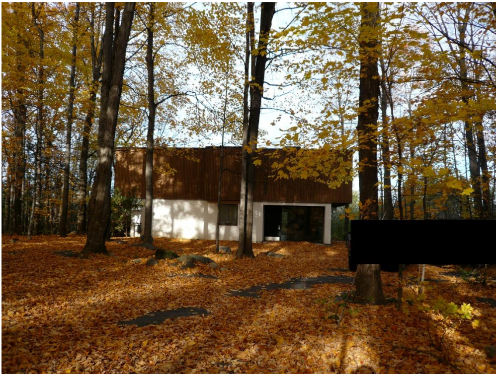
Front façade of house
