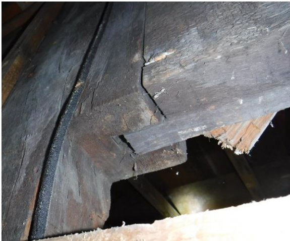
Figure 3: Post with Tenoned Timber
