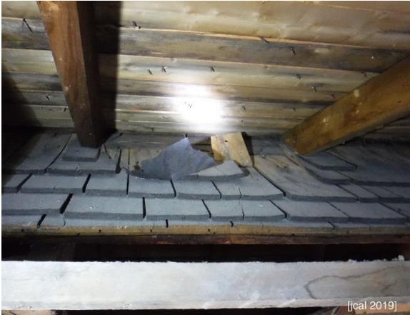
Figure 7: Dormer Rafters Bearing on Original Roof
