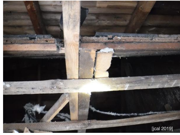
Figure 8: Cut Rafter End
