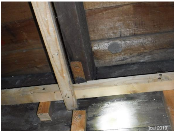
Figure 5: Connection of Floor Framing to Wall
