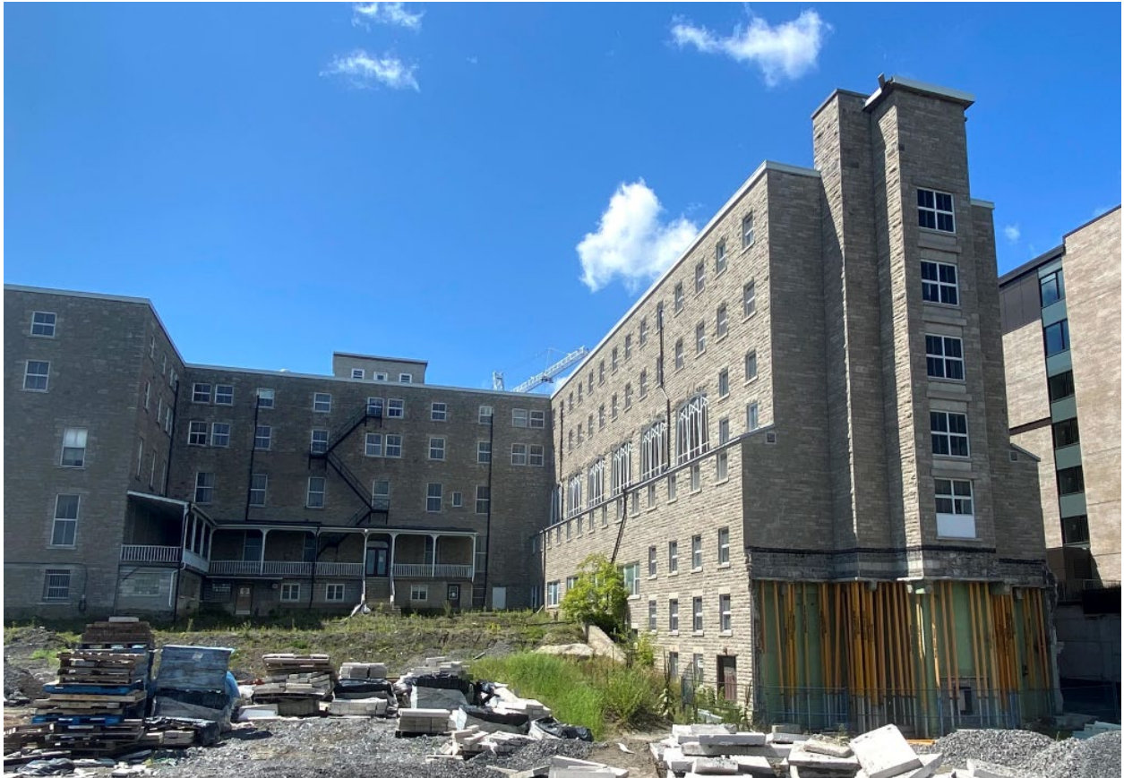
Chapel wing to be demolished, and porch to be removed
