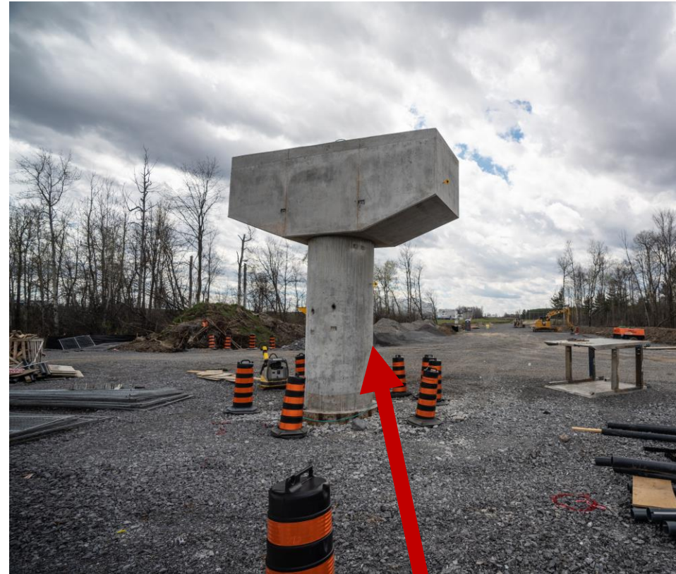
Uplands (west) substructure.
