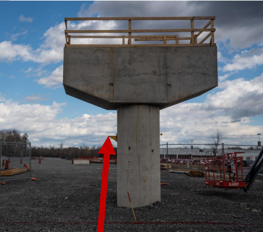
Uplands (east) substructure.
