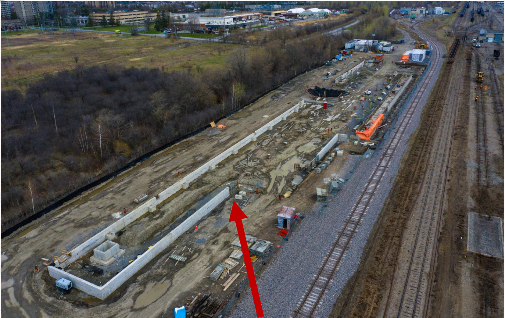
Pouring grade beams at the Walkley MSF.
