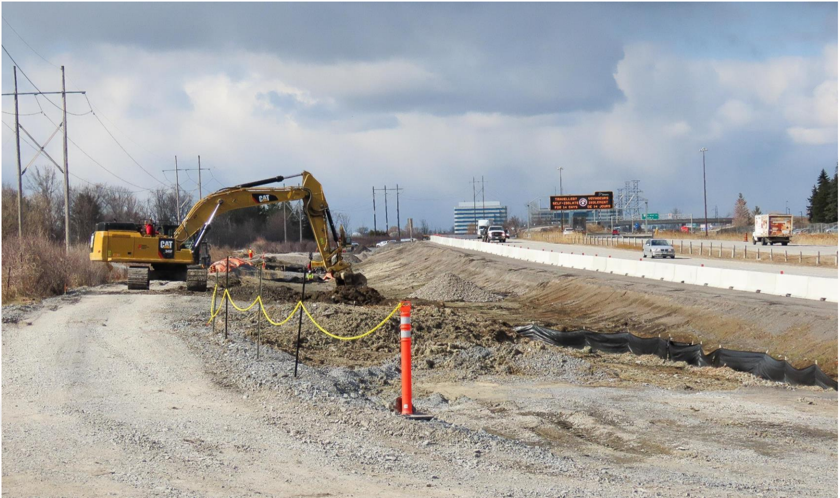
Roadworks on the south side of Highway 174, near Jasmine Crescent.
