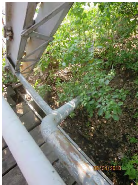
Photograph 52: Start of gas line at south end.
