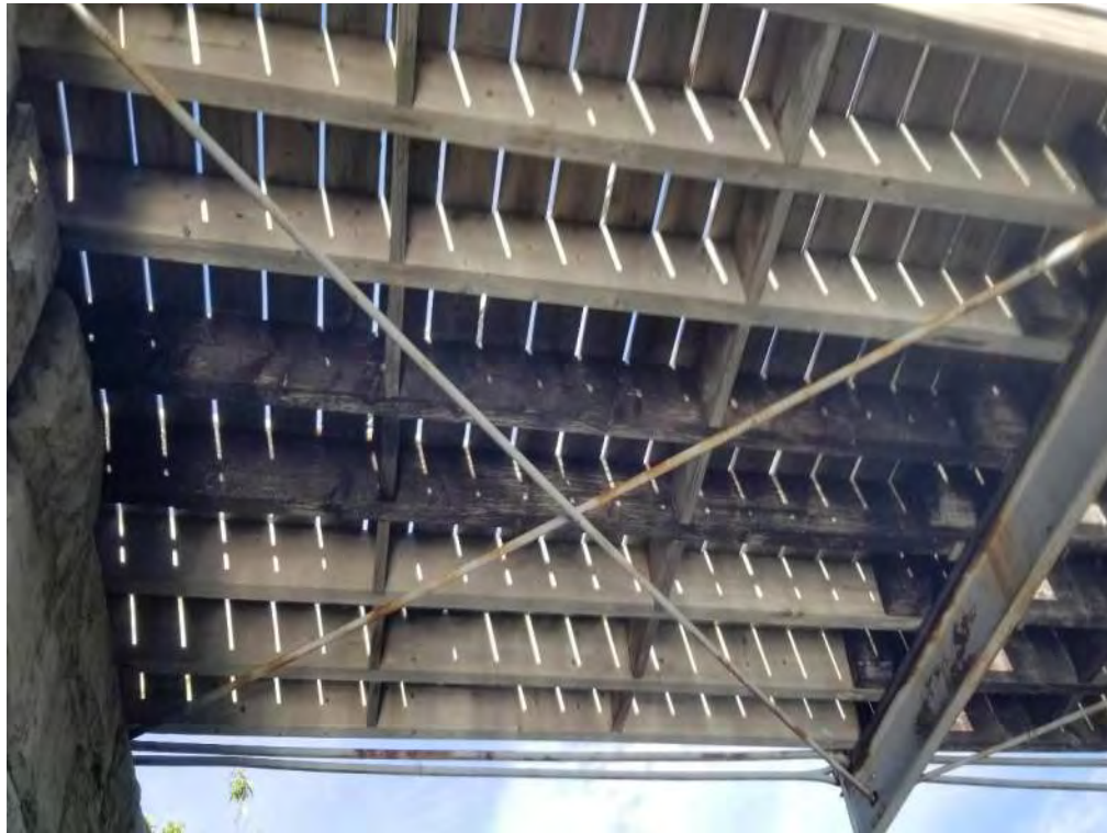
Photograph 29: Deck underside at pier. Note new stingers vs. original.
