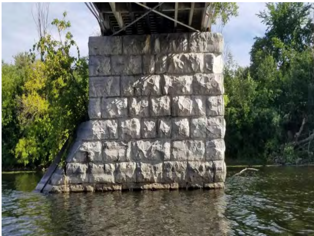
Photograph 46: North face of Pier.
