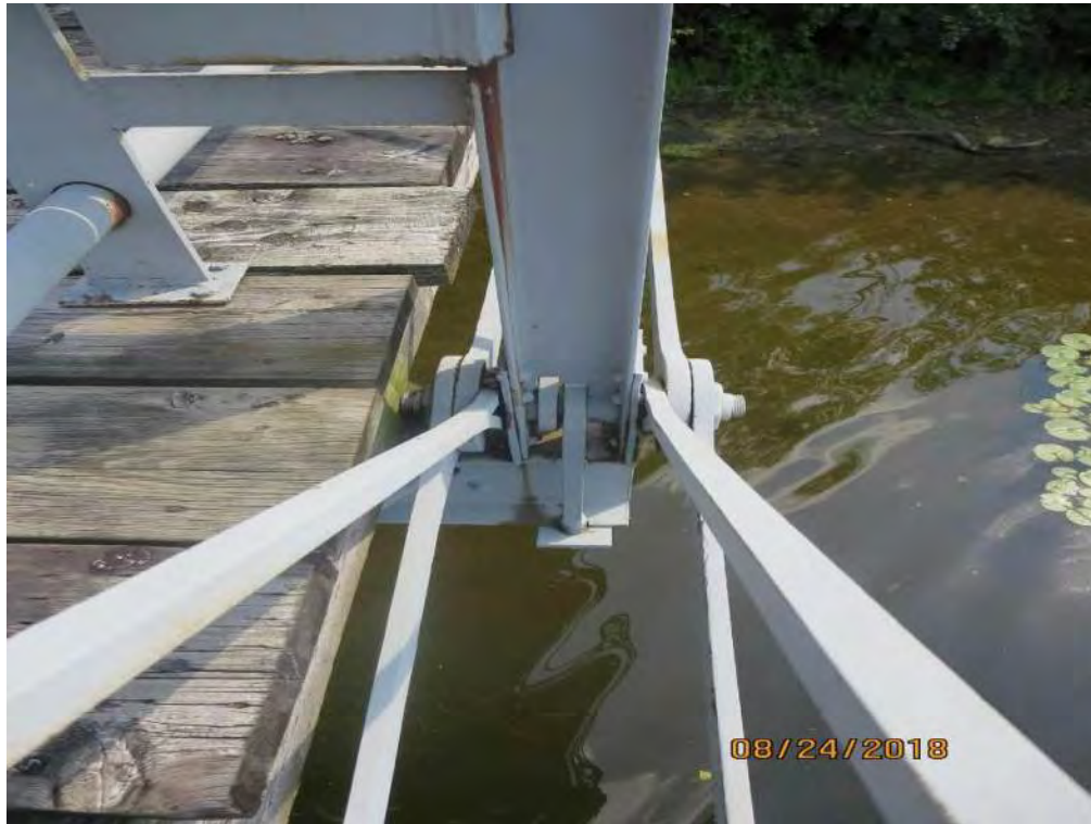
Photograph 15: Typical interior panel pin and hanger connection.
