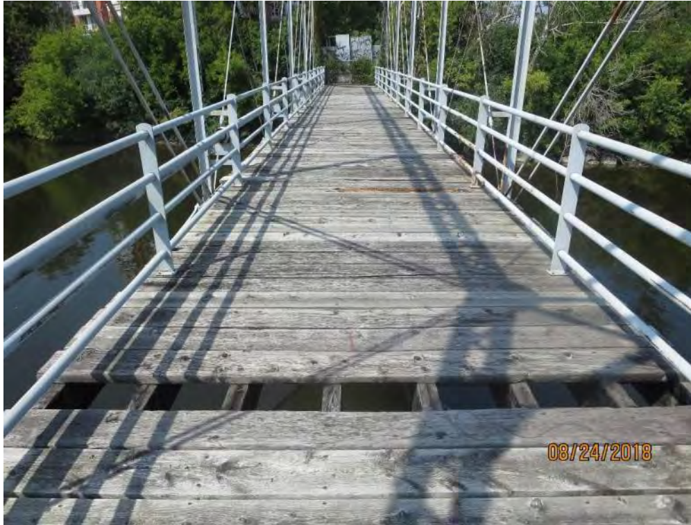
Photograph 23: Typical condition of deck.
