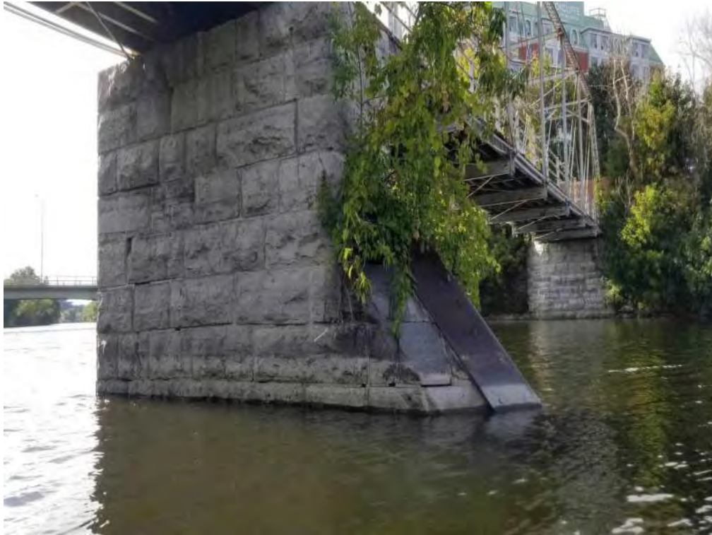
Photograph 45: South face of Pier.
