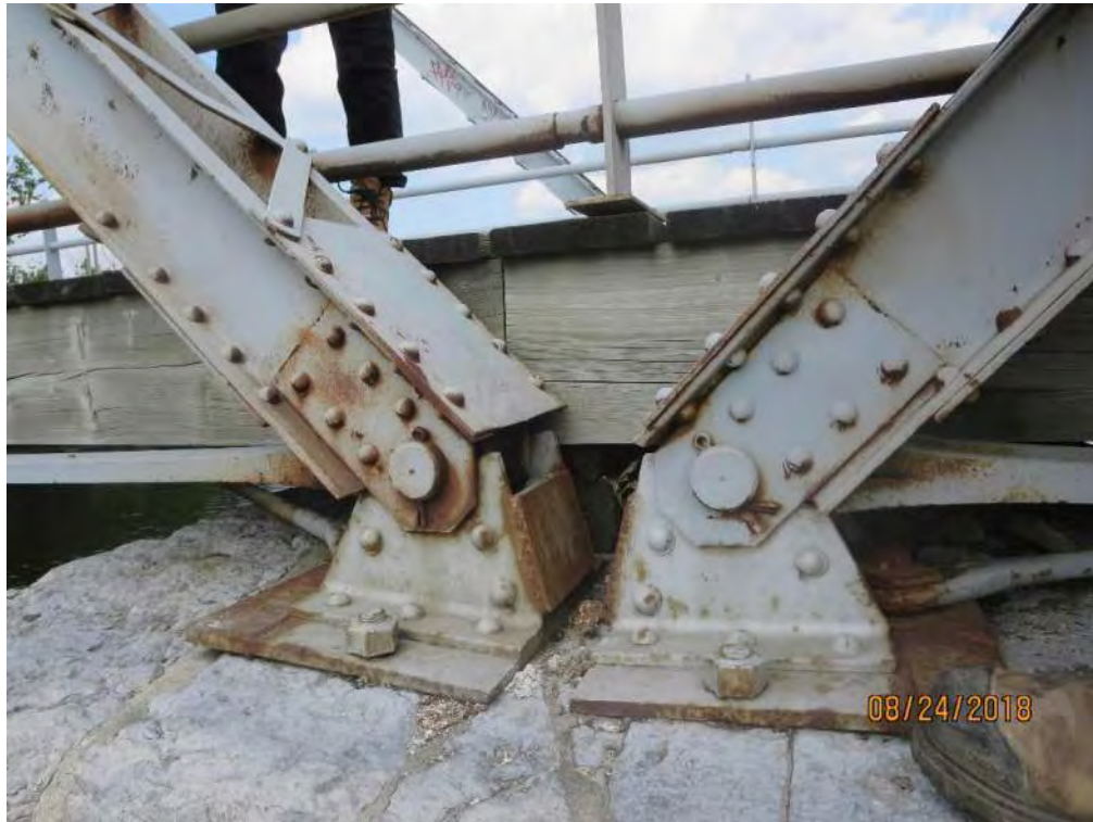
Photograph 39: Typical condition of Pier bearings.
