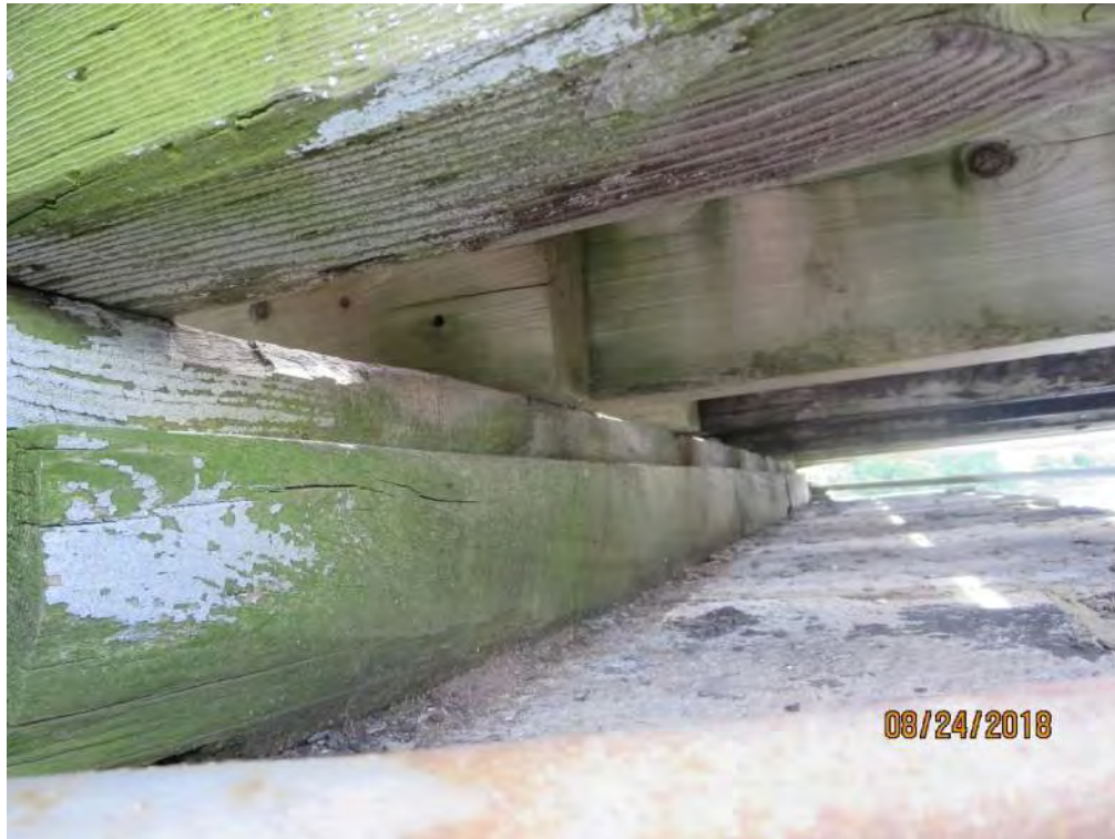
Photograph 47: Pier bearing seat.
