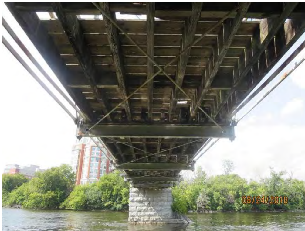
Photograph 28: Typical condition of underside of deck and cross bracing.
