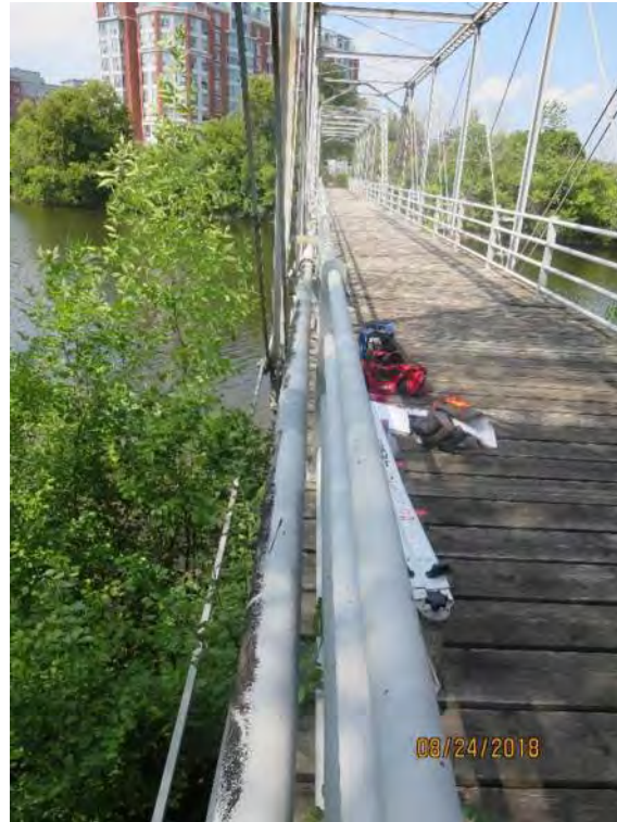
Photograph 51: Gas line on west side of deck.
