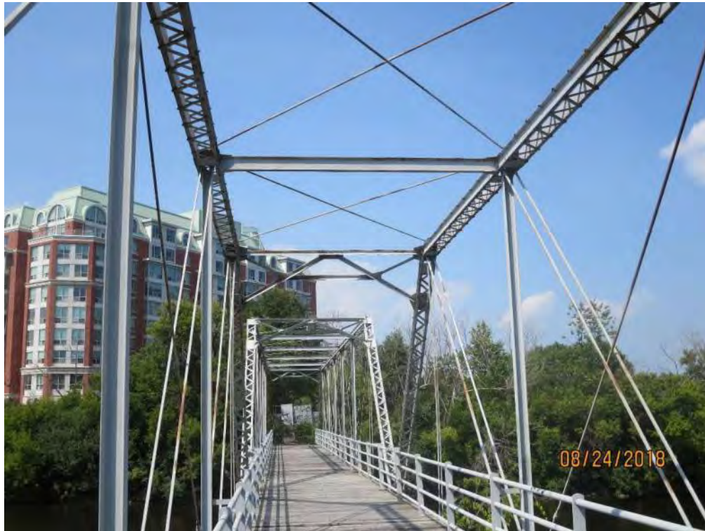
Photograph 5: Typical condition and general view of truss members.
