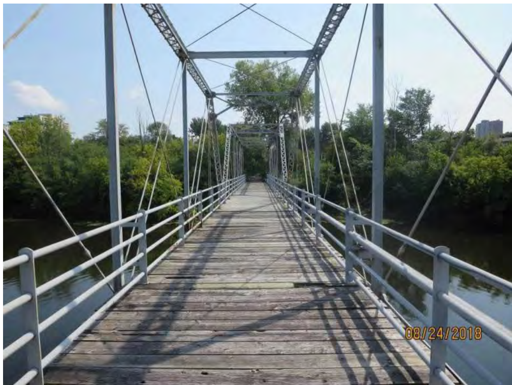
Photograph 4: Cross section of structure looking south at the pier.
