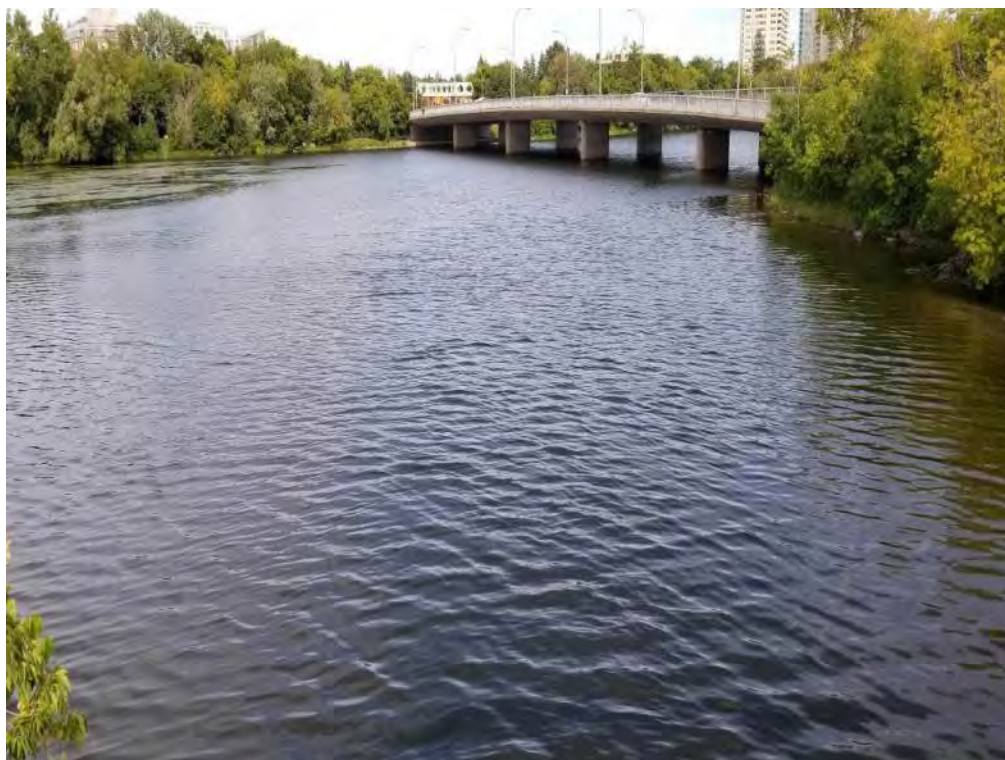
Photograph 50: General view looking east on structure.
