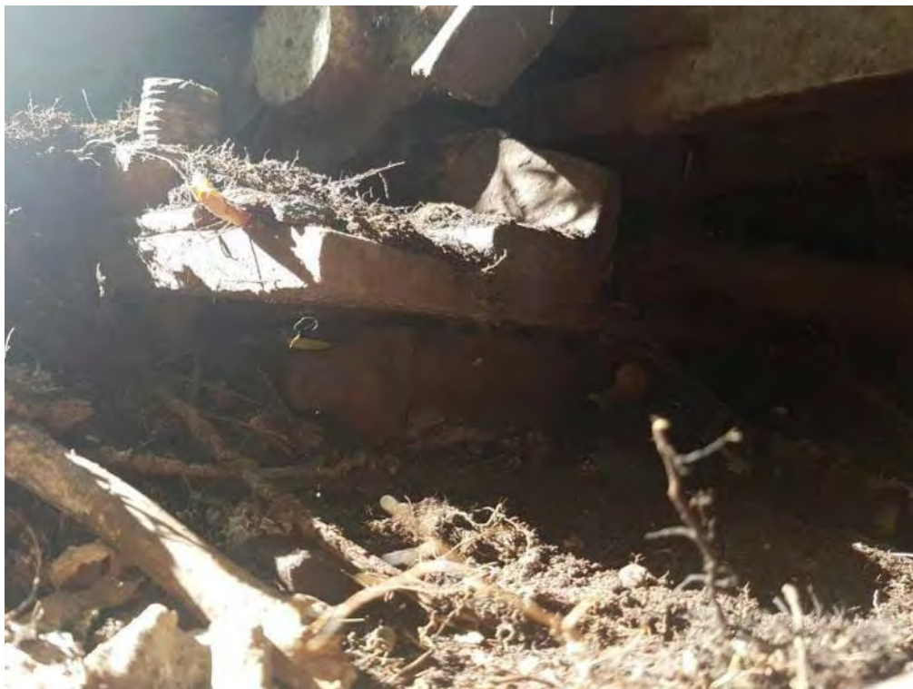
Photograph 37: Close up of Photograph 36.
