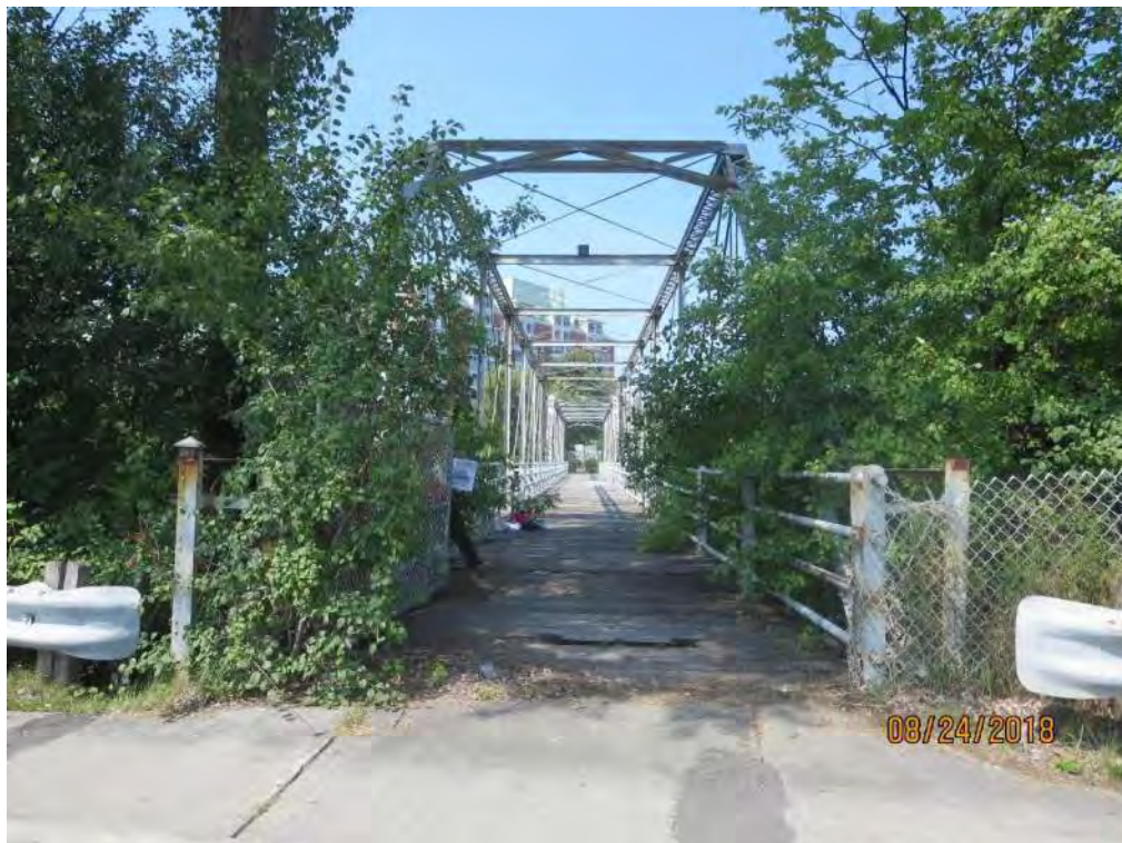
Photograph 2: South Entrance from St. Patrick Street
