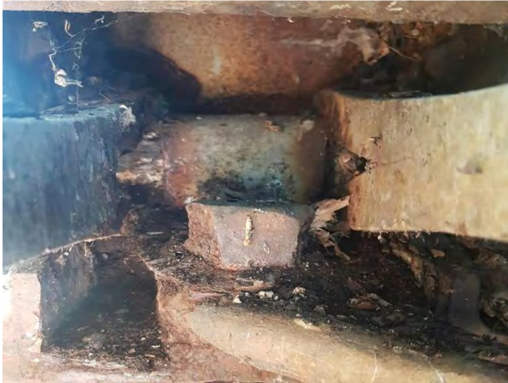
Photograph 21: Bottom chord connection at South Abutment (east side).
