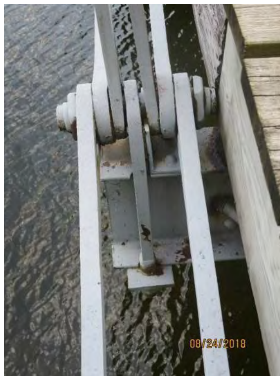
Photograph 14: Typical exterior panel pin and hanger connection
