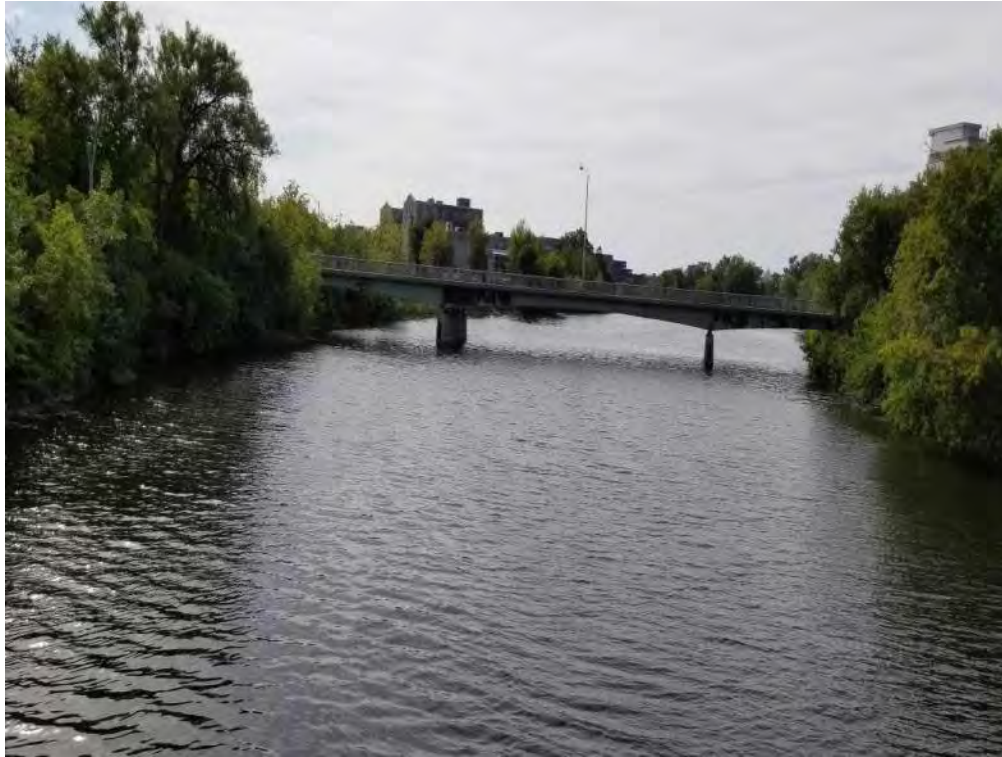
Photograph 49: General view looking west on structure.
