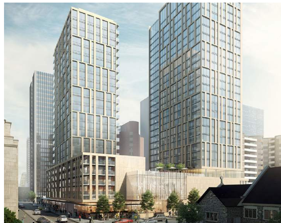
Fig. 24 Future multifunctional complex at 350 Sparks Street Source: www.wzmh.com/projects/350-sparks-street/
