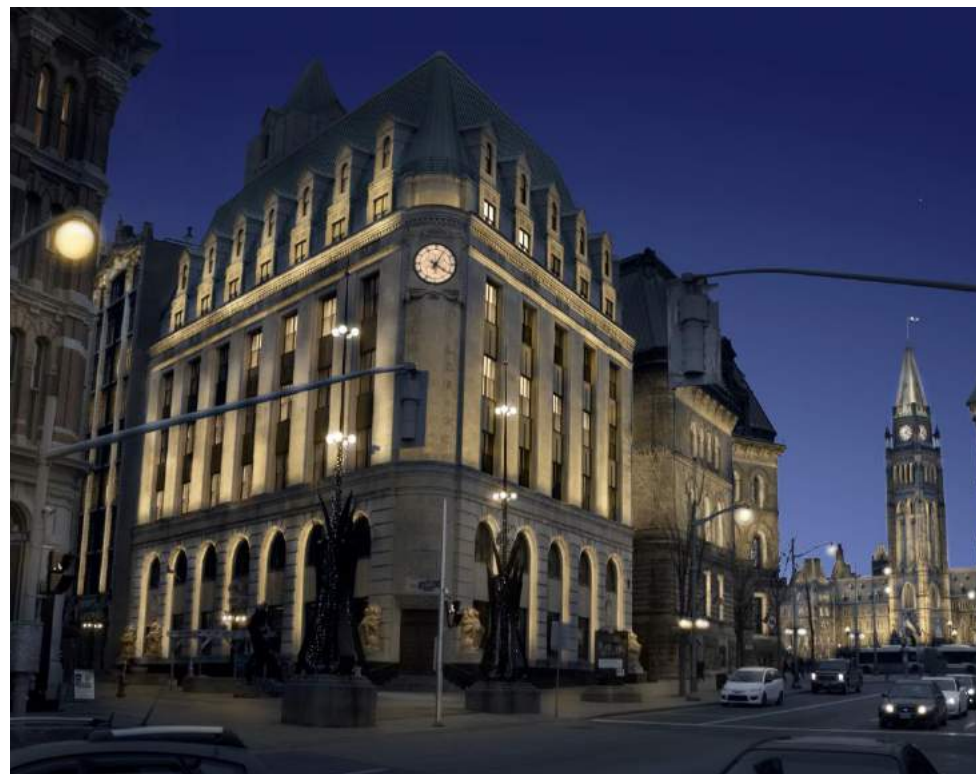
Fig. 62 View of Sparks Street and Elgin Street from the east side of Elgin Source: Parliamentary Precinct Exterior Lighting Master Plan, 2015
