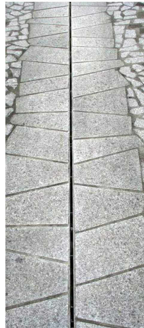
Fig. 142 Stormwater slot drain in paving Source: www.landezine.com/st-flour-pavement-by-insitu-landscape-architecture-01.jpg
