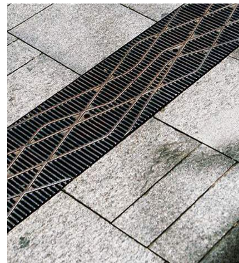
Fig. 140 Technical trench with decorative cover Source: www.landezine.com/index.php/2013/10/pitt-street-mall-by-tony-carro-architecture/
