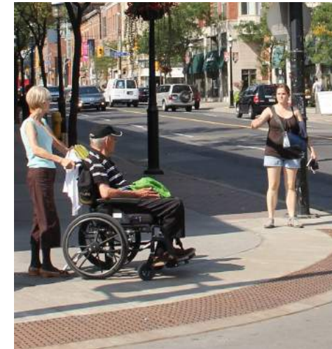
Fig. 103 Tactile Walking Surface Indicators Source: www.toronto.ca/services-payments/streets-parking-transportation/walking-in-toronto
