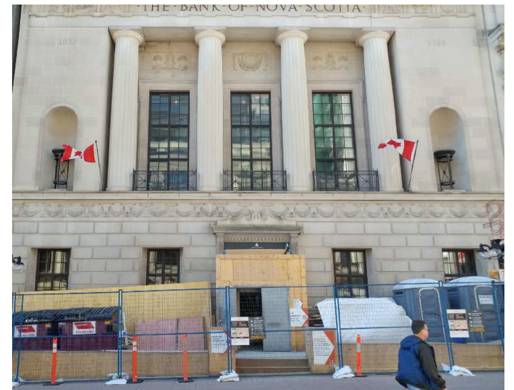
Fig. 25 Construction at the Bank of Nova Scotia Building Source: Vlan + civiliti
