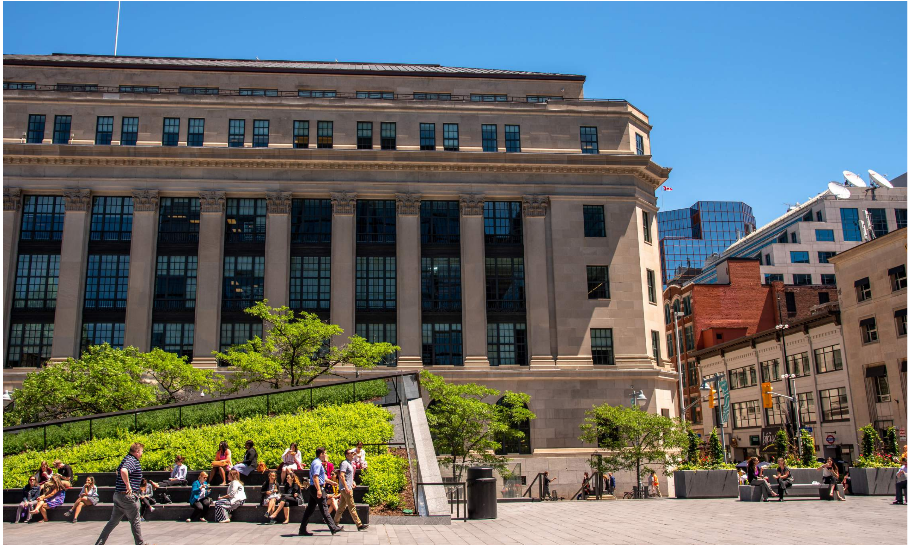
Fig. 53 The Bank of Canada Museum Plaza and the classified heritage Wellington Building in the background Source: City of Ottawa
