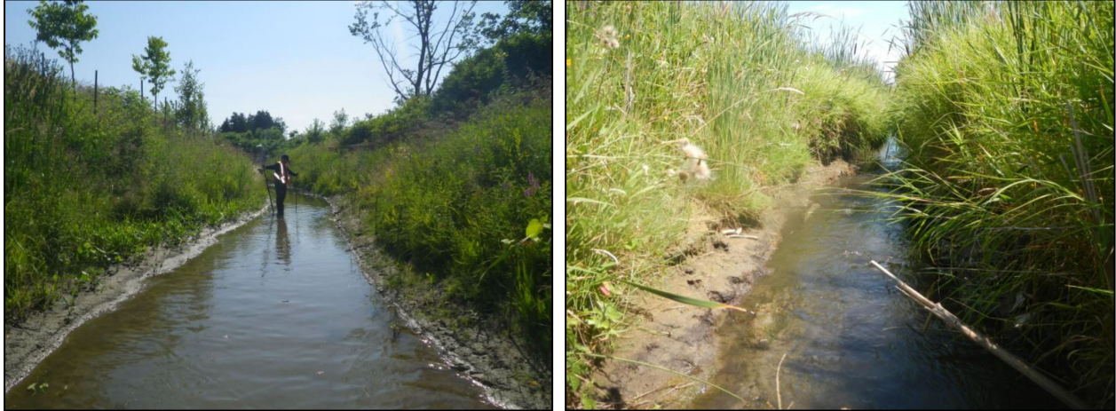
Figure 2.2. Channel in Straightened Reach 3 (on the left); Failure of Creek Bank from Scour in Reach 6 (on the right)
