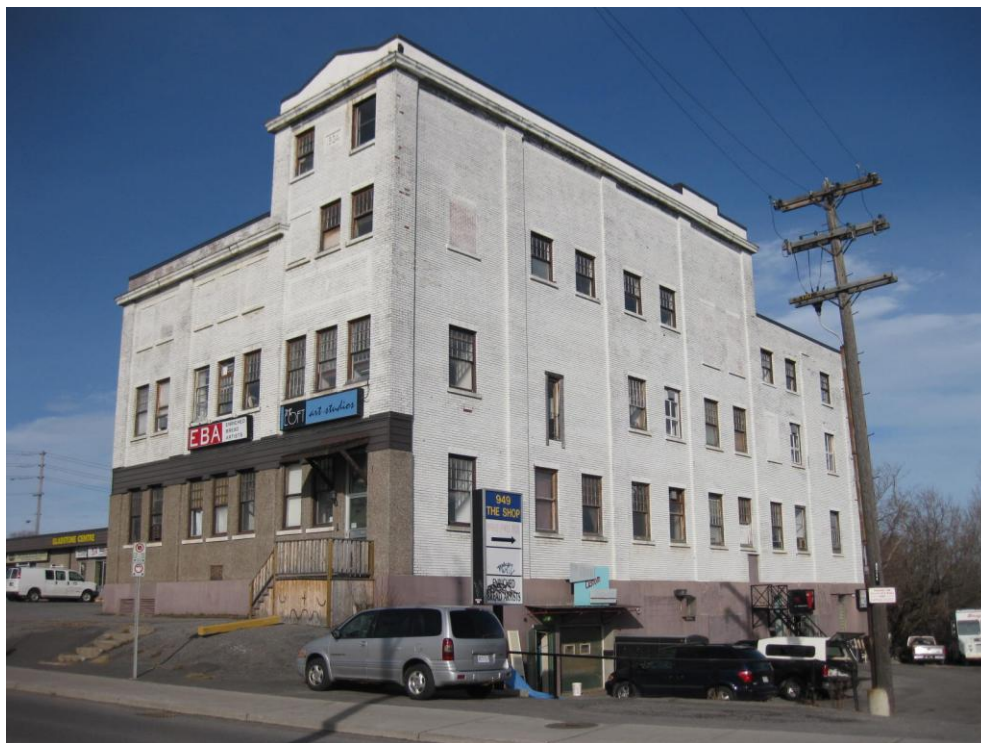
Exterior photo 2010, prior to removal of parapet from storm damage
