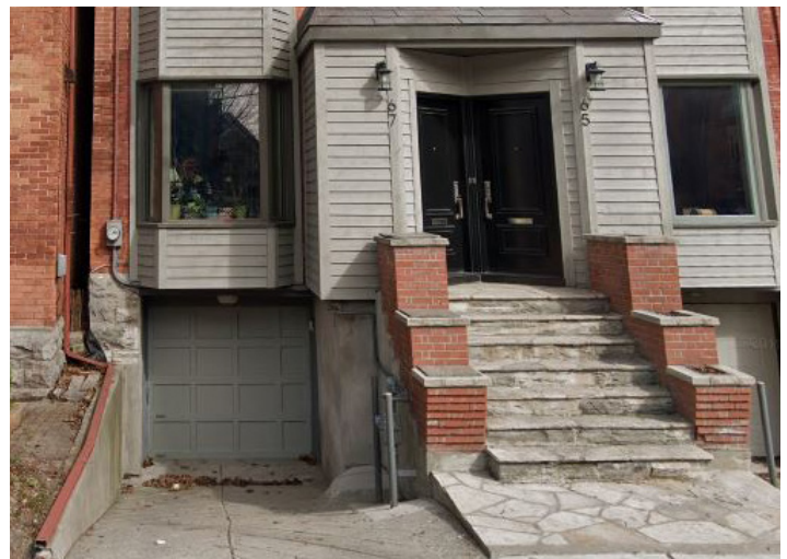
Figure 18: Example of a below grade garage facing the street
