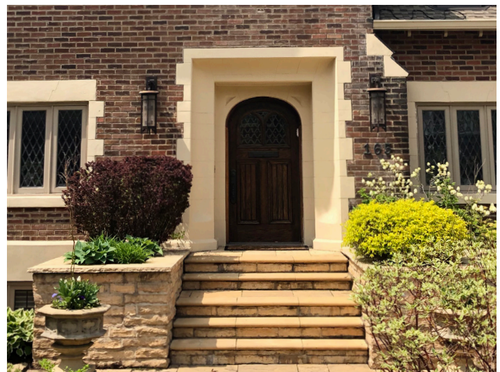
Figure 7: Example of historic elements of door openings
