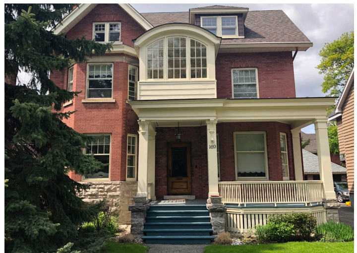
Figure 15: Example of an enclosed upper porch.
