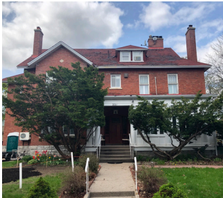
Address: 640 Lyon Construction Date: 1909 Architect: John Pritchard Maclaren Note: 221 Clemow
